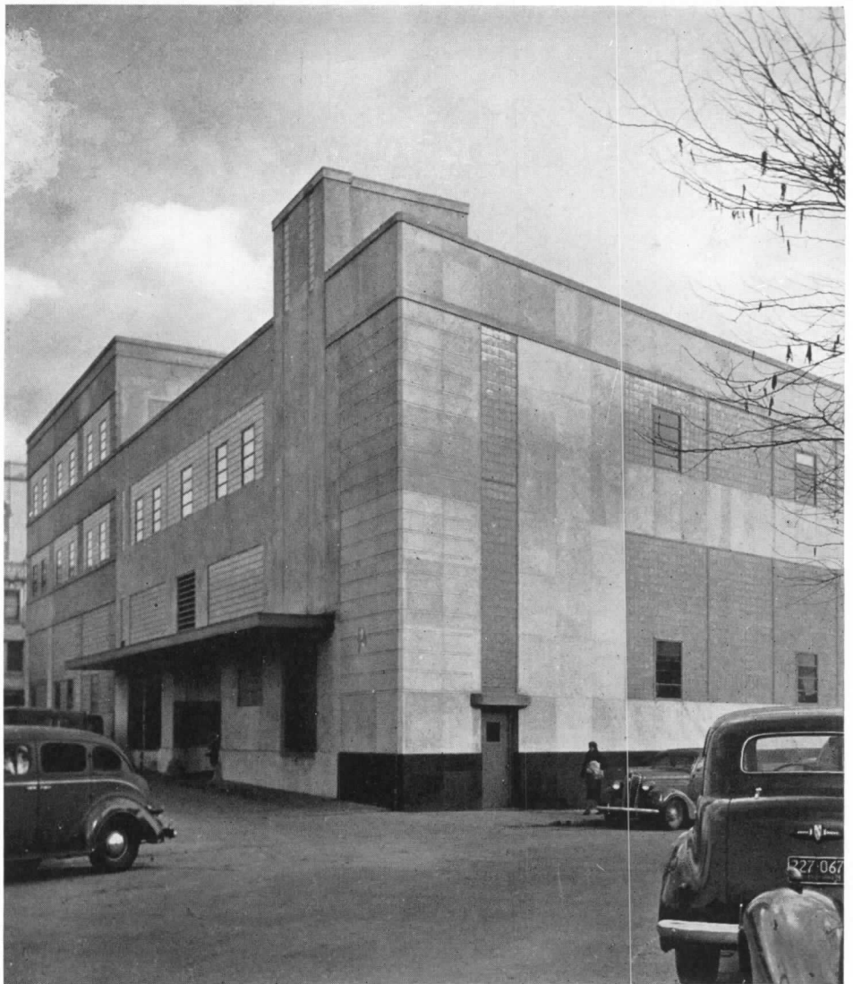
REAR VIEW. Advantage was taken of the site slope to the rear for simplifying the handling of stores of newsprint and ink, a very considerable item. From the truck-bed-high loading platform near the rear of the building, paper goes to the basement on an electrically operated paper drop. Thereafter it is handled horizontally on dollies running on trackage sunk below basement level (see basement floor plan) either to storage room or reel room from which the press is serviced. Space is provided for a month's supply
