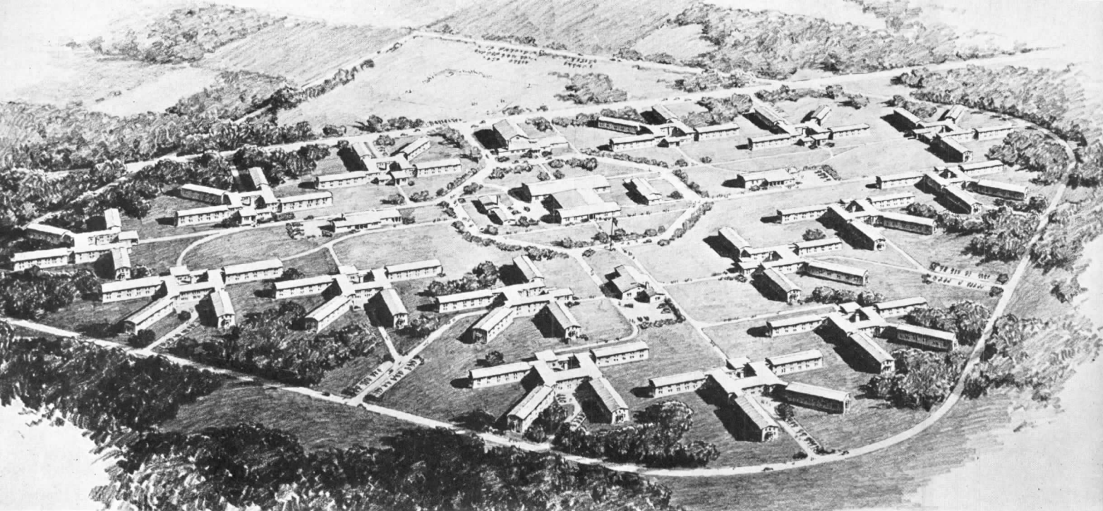
Air view of dormitory group planned to house approximately 3,000 workers
