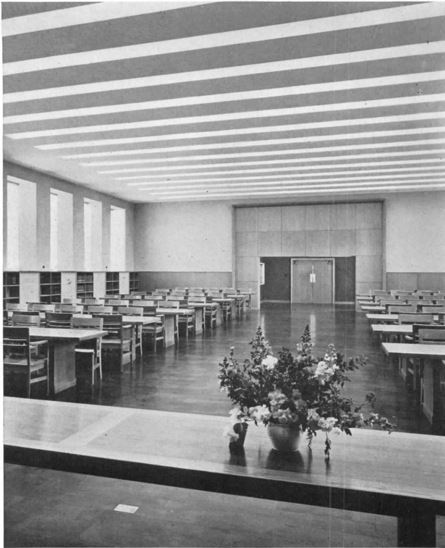
LIBRARY. Acoustical ceilings; fluorescent light, flush mounted
