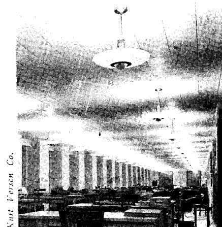
Plastic luminous-bowl ceiling fixtures
