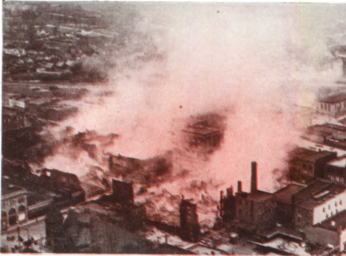
Not a bombed area - 17 buildings destroyed by fire in the business district of a mid-western city.
