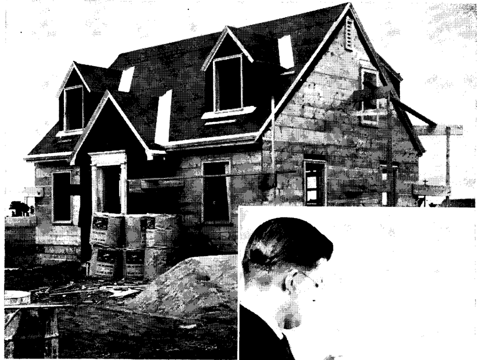
Framing up one of the Test Houses— Balsam-Wool on the Job. →
