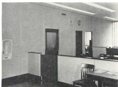
Movable partitions and acoustic ceiling
