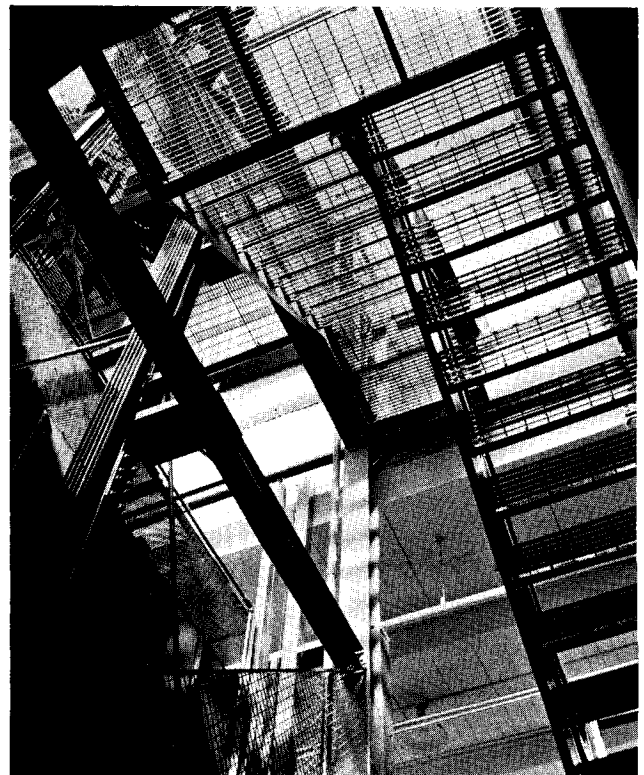
Above (and below) : The railroad siding, running through the rear of the building, made it necessary to use a free standing fire escape. Note the simple method of supporting it—one channel column. Right: in the two-story scheme small parts are made in the light machine shop on the second floor and transferred by means of the elevator to the main floor for assembly and shipping. The combined stair and elevator shaft is left open, with open mesh partitions and stair treads, to get daylight into the shaft from a skylight in the roof
