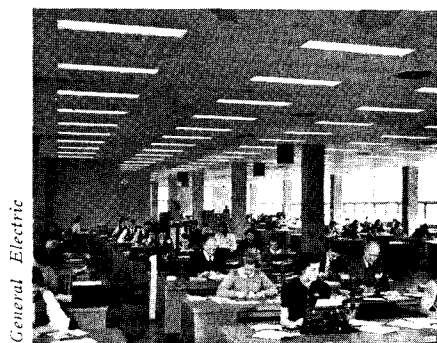
Flush-mounted troffers on 6 ft. centers
