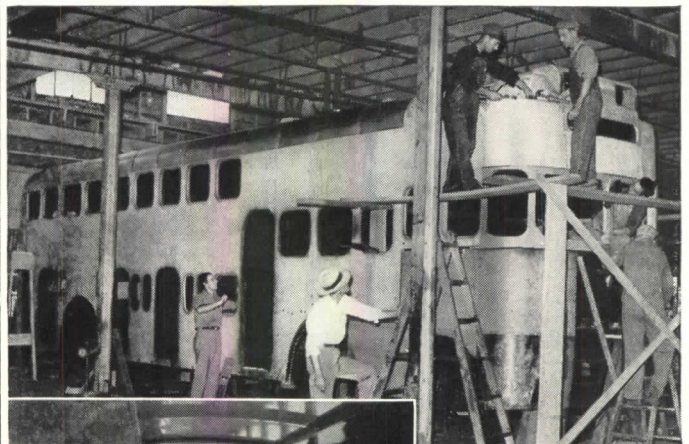
(At top of page) One of Santa Fe Trailways' smart new 117-passenger Victory Liners. The exterior, interior, partitions and floors are built of Douglas Fir Plywood. Now under construction is a 150-passenger all plywood Victory Liner.
