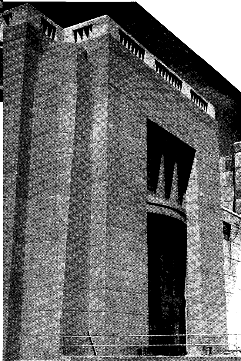
Rustication lines give scale to mass walls of Santee-Cooper powerhouse. Building designed by Harza Engineering Co., Chicago. Built by Central Engineering Co., Davenport, Iowa.
