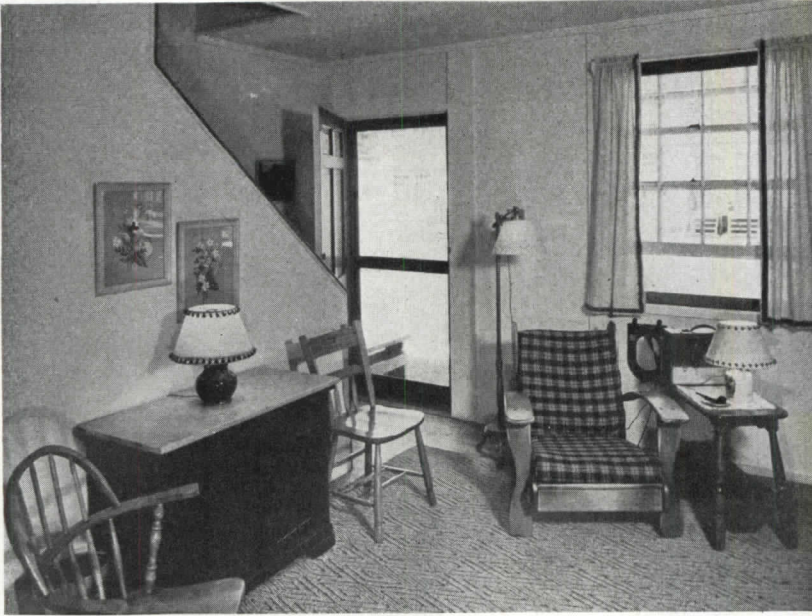
Interior views of 35th Street Houses, the first of the prefabricated demountable war housing projects of the National Capital Housing Authority. The plans below were also used for Monroe Street
