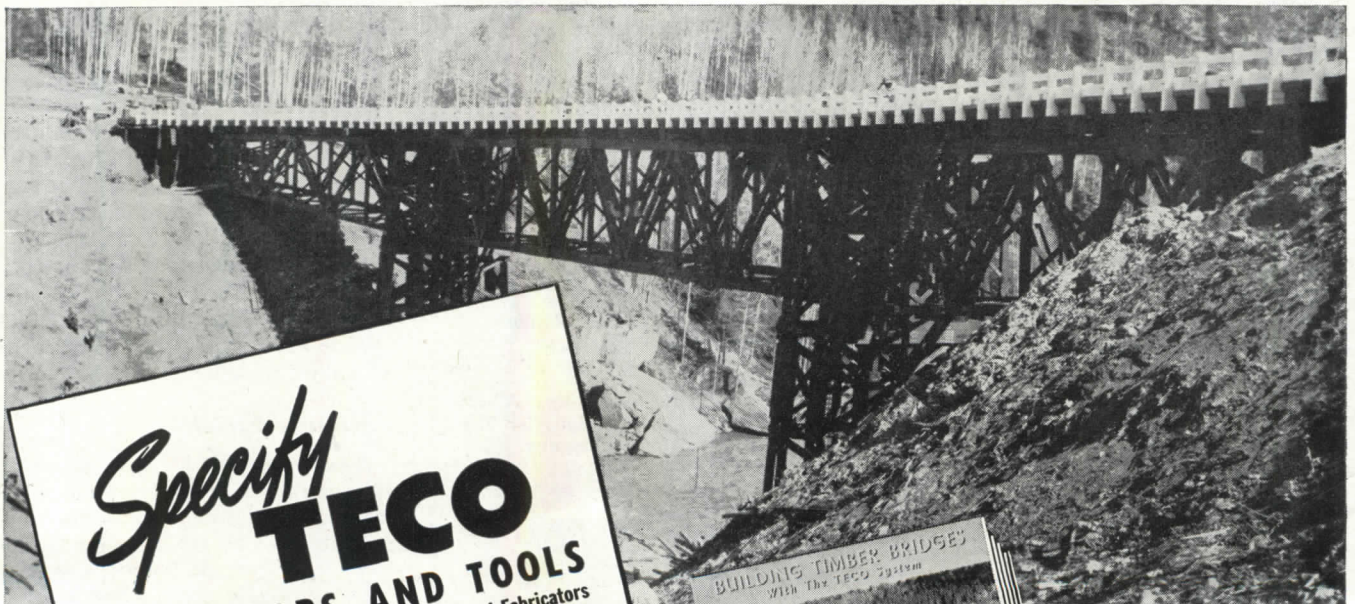
THE KISKATINAW RIVER BRIDGE, one of the major crossings on the Alaska Highway, designed by the U. S. Public Roads Administration. The timber superstructure was prefabricated and pressure-cresoted by the Canada Cresoting Co. The Timber Connector System was used.
