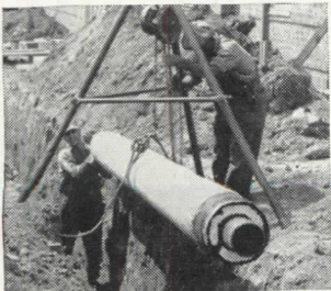
Section of Ric-wil prefabricated insulated steam conduit being lowered into shallow trench for steam connection to a new apartment at Shaker Square.
