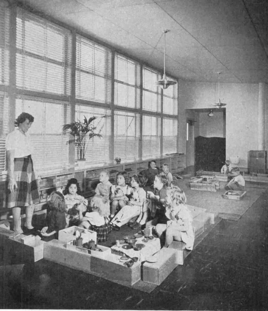
Kindergarten room in the elementary school building, left and immediately below. Bottom: a typical classroom, showing bilateral lighting from clerestory windows
