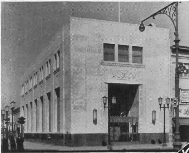
South Brooklyn Savings Bank (Brooklyn, N. Y.), Dudley E. Soper, Architect. Child & Scott-Donohue Inc., Heating Contractors. BOILER PLANT — 2 — H. B. SMITH No. 34 "MILLS" BOILERS.
