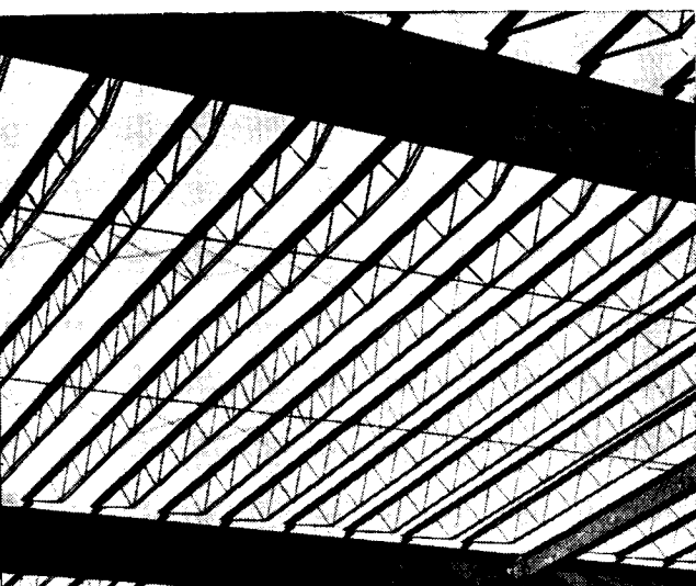
Beauty of construction is made possible by Ceco steel joists. No special skill or equipment needed in placing them. They are easily moved into position and quickly spaced. After bridging, floor and ceiling are installed.
