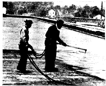
Faster roof-coating by cold-spray method
