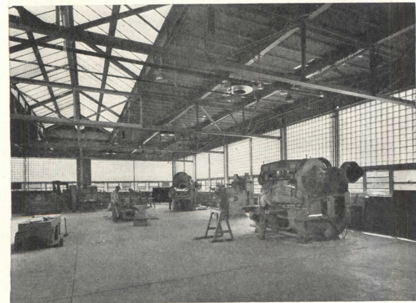
Ceiling-high Insulux panels distribute daylight across broad work areas, cut off distracting views. Clear windows furnish ventilation and vision out. Insulux Glass Block has proven advantages in all classes of construction.
