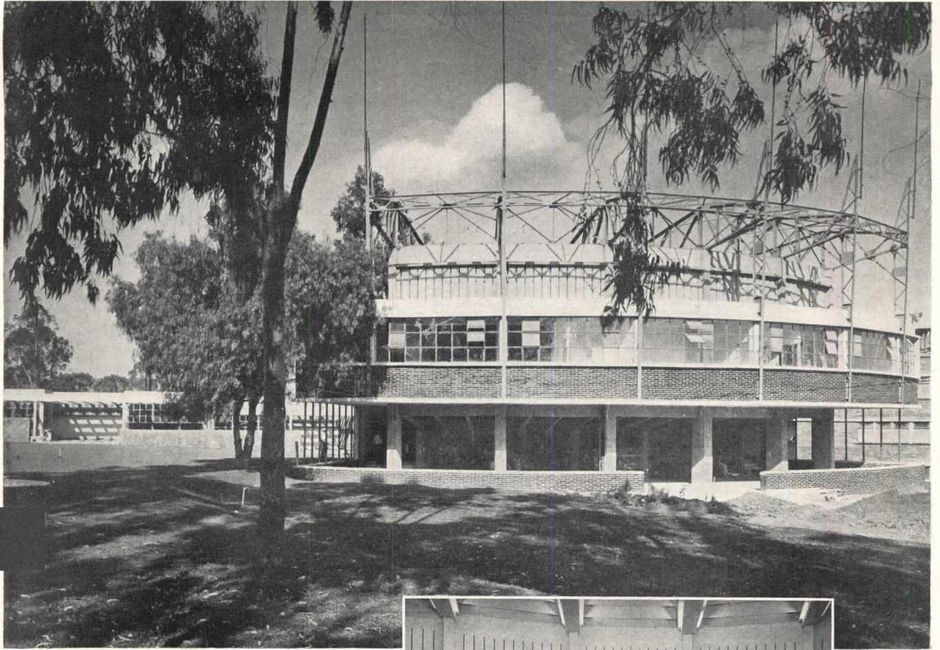
10. The auditorium is an interesting example of an exoskeleton in which the exposed structural elements constitute major design forms and produce unusual shadow effects. Problems of weather-tightness and increased maintenance costs are frequently deterrents to more universal acceptance of such structures
