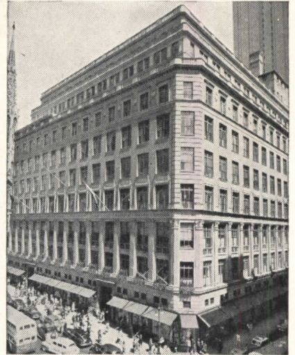
SAKS & COMPANY, Fifth Avenue, New York, N.Y. Built 1924. Architect: Starrett and Van Vleck. Heating Contractor for original installation: Gillis and Geoghegan. Heating Modernization 1944 by Contractor Thomas J. Dorsey, Inc.
