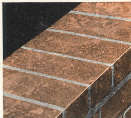
This completely fills the joint.
