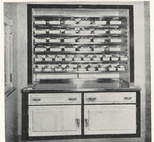
Recessed cabinet in maternity department. Upper section open and fitted with adjustable stainless steel shelves for holding mothers' treatment trays.
