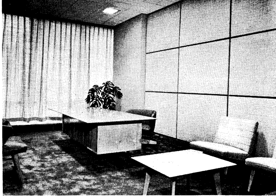
Another executive office. One wall is paneled and "padded" with acoustical blankets covered with black and white Fiberglas-wool fabric, close-up at left. Ceiling is Fiberglas acoustical tile (Securitee system)
