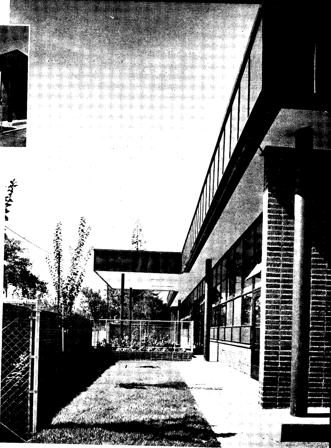
In the two small top views, the awnings may be seen pulled down—the architects say this saves expense of air conditioning. At right they are seen rolled up into the soffit of the overhang. Awnings are tan, pipe columns vermilion, overhang band copper-faced. Walled-in front gardens (right) give executives a pleasant outlook; chain link fences at ends let breezes through. For planting plan, back garden, see p. 90
