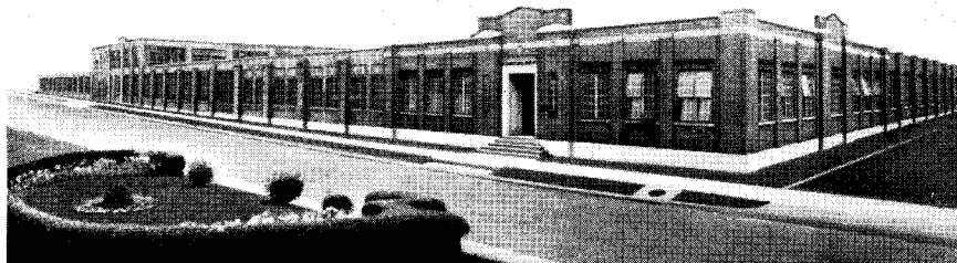
Main office and factory of Jamestown Metal Corp.
