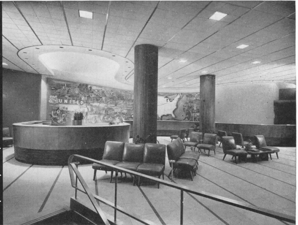
United Air Lines Ticket Office, Chicago. Multi-Vent Panels completely concealed by metal acoustical ceiling.
