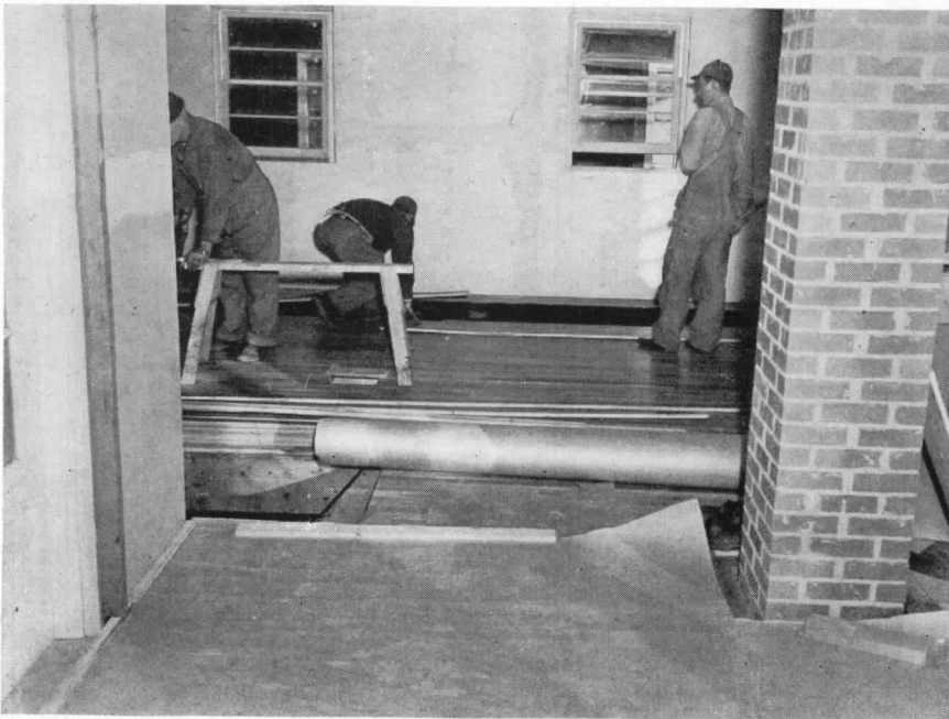
Above and below: finished flooring is laid before partitions are erected, and protected with one layer of wrapping paper and one of sisalkraft, held down by batten strips
