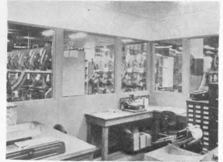
Thermopane, well known as a heat insulator, is now used to eliminate noise
