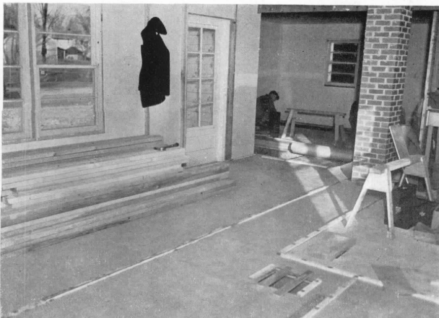
Above and below: finished flooring is laid before partitions are erected, and protected with one layer of wrapping paper and one of sisalkraft, held down by batten strips
