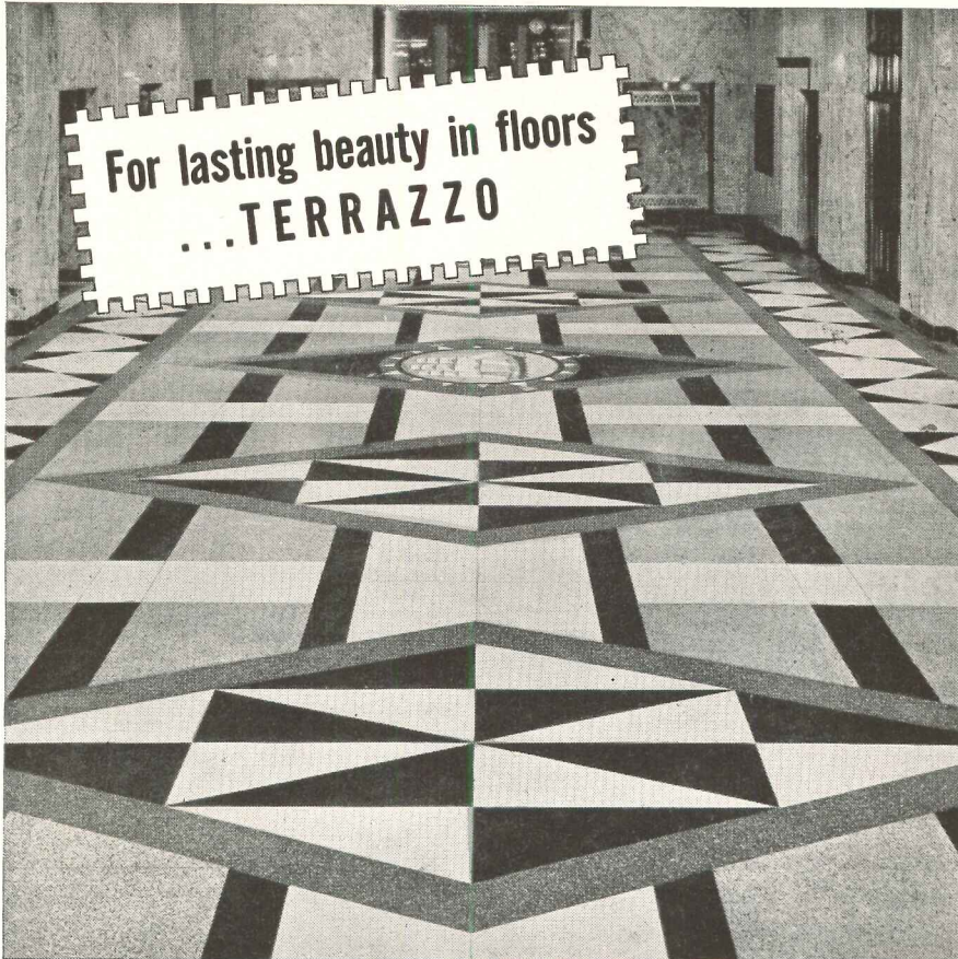
Boston University's Administration Building lobby. Architect, Cram & Ferguson; Terrazzo Contractor, De Paoli Mosaic Co.; both of Boston
