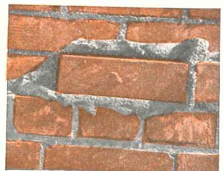
So that the mortar oozes out at the top of the joint.
