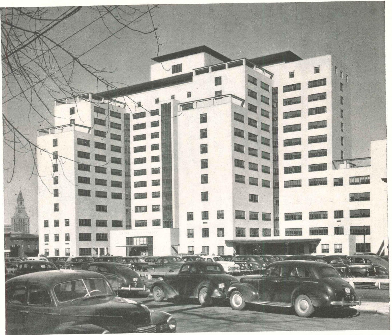
Architects: Coolidge, Shepley, Bulfinch and Abbott, Boston. General Contractor: George A. Fuller Co., Boston. Steel Fabricator: Utica Structural Steel Co., Utica, N. Y.
