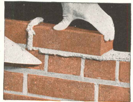
So that the mortar oozes out at the top of the head joint.
