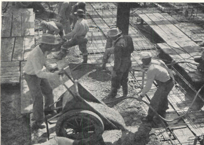
Left: pouring lightweight pumice aggregate in the construction of floor slabs and fireproofing the main girders and tie beams; mix is placed with help of pneumatic vibrators. Right: secondary beams and interior columns are fireproofed with vermiculite in plaster
