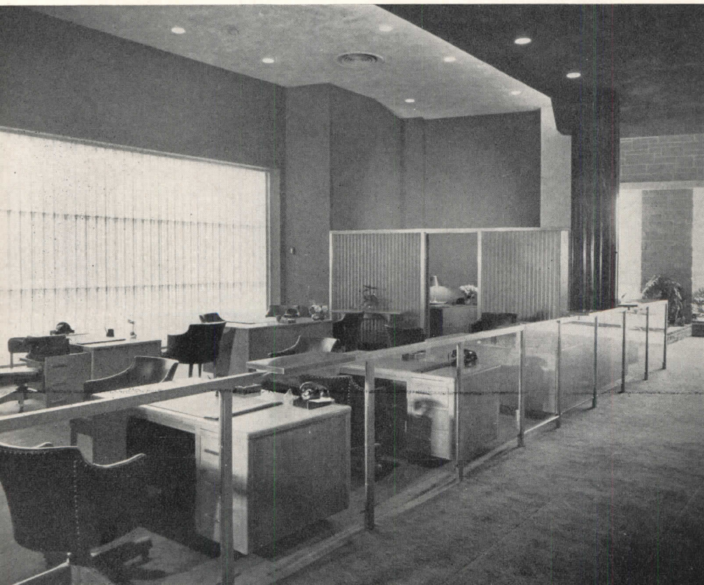
Above: view through the bank from main entrance to parking lot. Columns are green Verde Antique marble. Ceiling is sprayed asbestos to increase acoustical absorption; center portion is 2 ft. lower than side panels, permitting continuous longitudinal fluorescent light troughs. The drop ceiling also has rectangular light troughs, and flush floods are widely used
