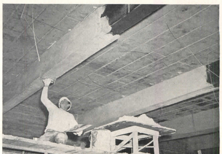
Left: pouring lightweight pumice aggregate in the construction of floor slabs and fireproofing the main girders and tie beams; mix is placed with help of pneumatic vibrators. Right: secondary beams and interior columns are fireproofed with vermiculite in plaster
