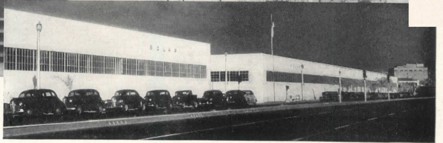
82,535 sq. ft. of Cemesto, clipped to steel beams, provides insulation, light-reflecting interior finish, and great strength with light weight—applied as structural roof deck on the Solar Aircraft Company's new plant, San Diego, California.
