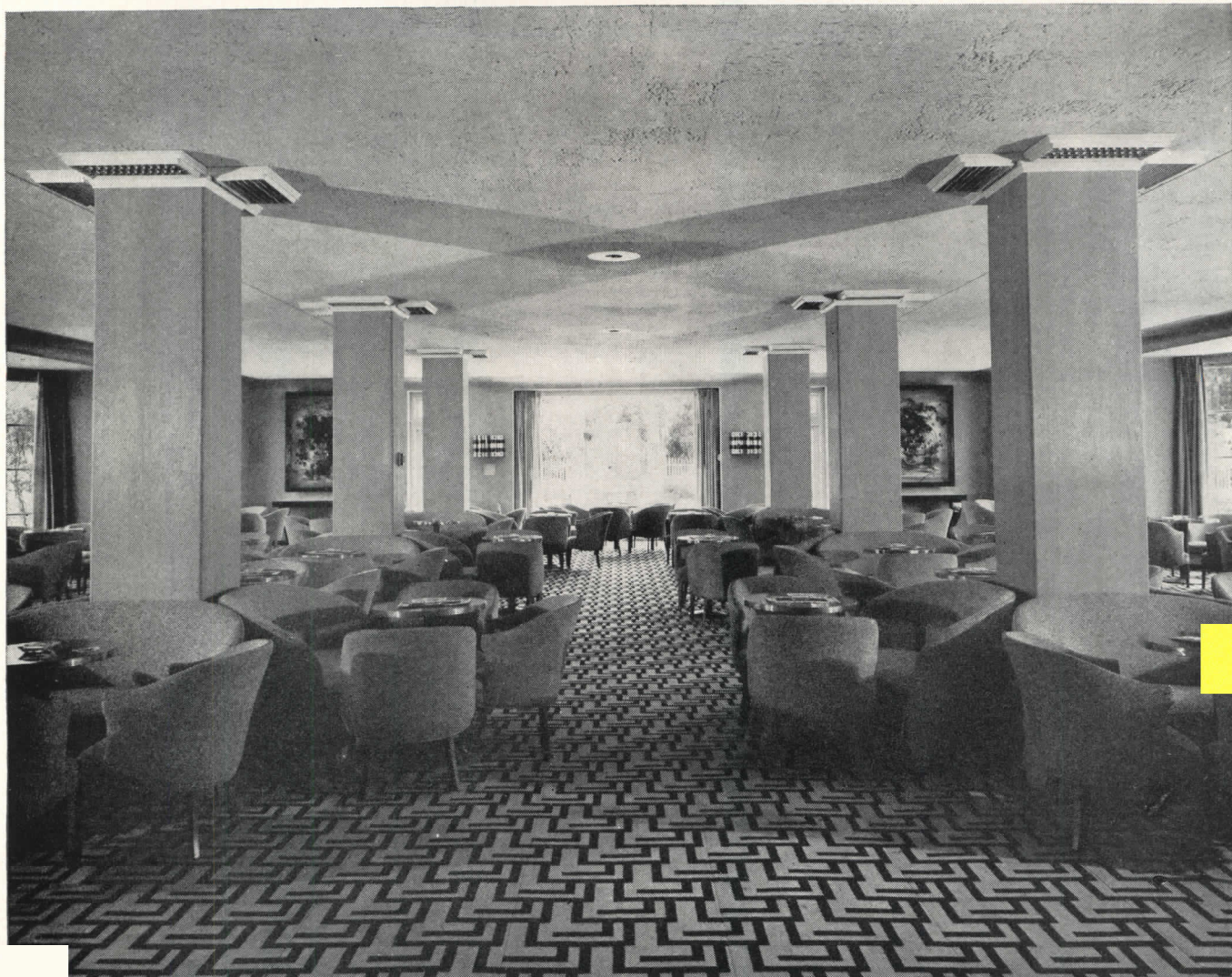
Versatile Agitair Type R's placed around columns blend perfectly with surroundings and provide 100% air distribution in the Old White Club of The Greenbrier.
