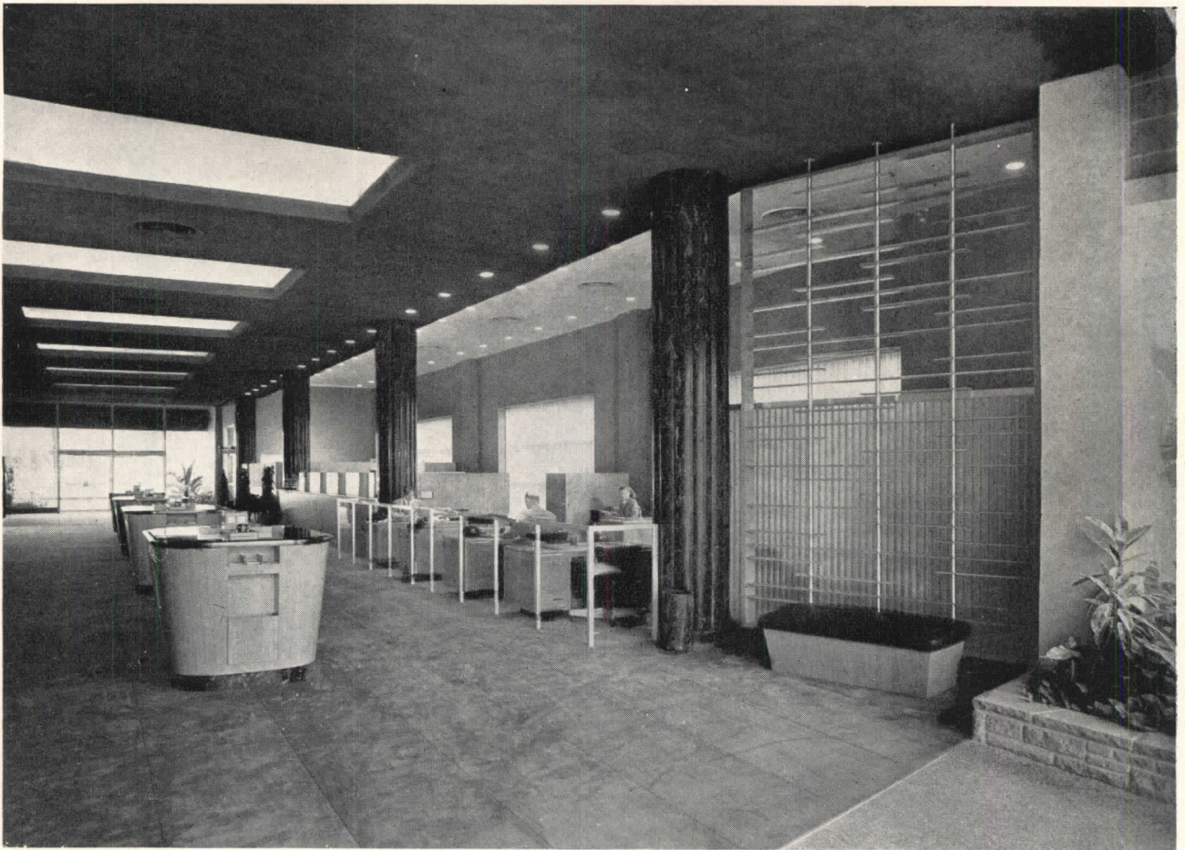
Above: view through the bank from main entrance to parking lot. Columns are green Verde Antique marble. Ceiling is sprayed asbestos to increase acoustical absorption; center portion is 2 ft. lower than side panels, permitting continuous longitudinal fluorescent light troughs. The drop ceiling also has rectangular light troughs, and flush floods are widely used
