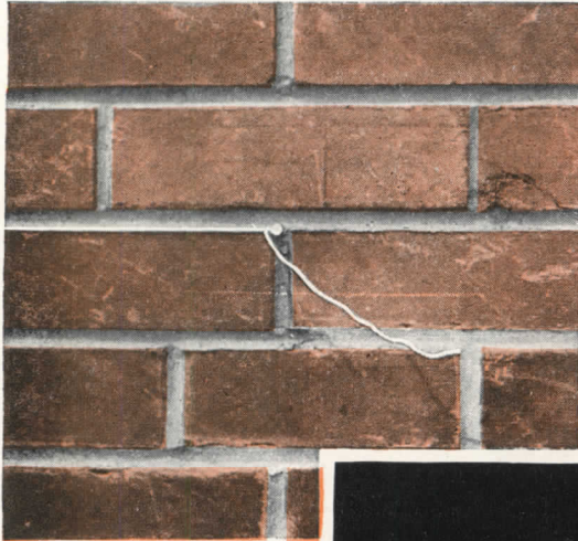
When a nail or line pin is used, the hole should be plugged with mortar as soon as the nail is removed.
