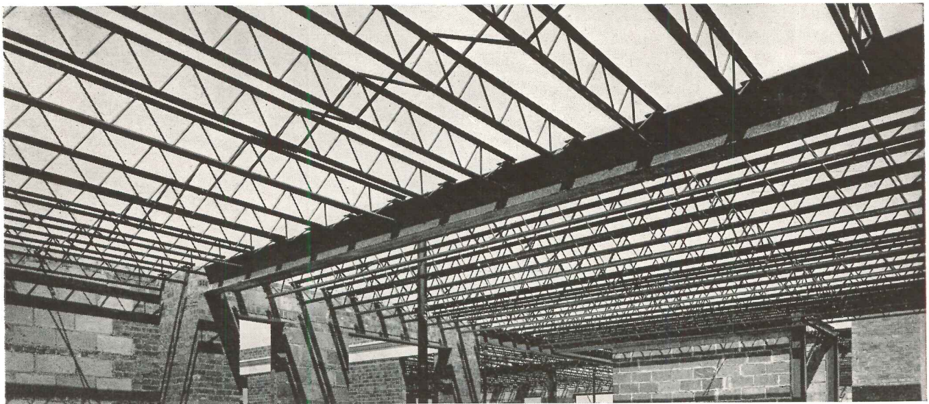
Construction scene, taken during erection of apartment buildings above, showing Bethlehem Open-Web Joists in place.
