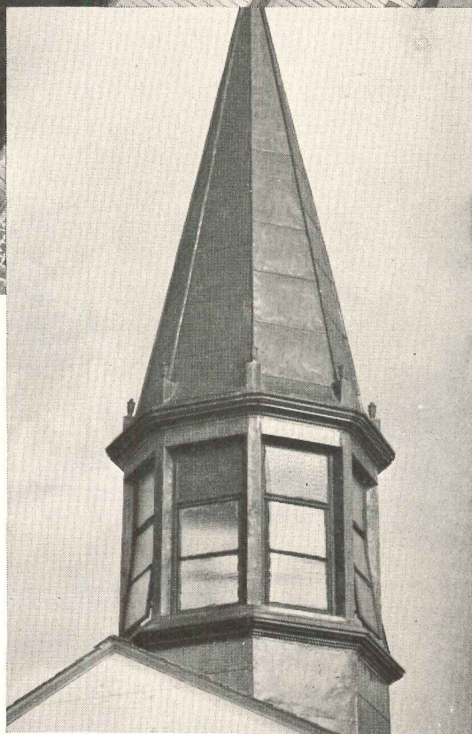
NEW CHAPEL OF LATTER DAY SAINTS, CHARLOTTESVILLE, VIRGINIA. J. H. SMITH, ROOFING CONTRACTOR
