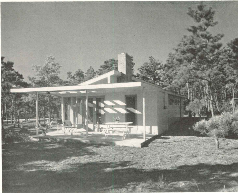
The east terrace-porch is frequently used for dining, served through the utility room. Below, a broad roof overhang on the south side shields the living and bed rooms from too much sun or rain and the pines provide shade for outdoor living. Exterior, vertical T & G local pine, painted white
