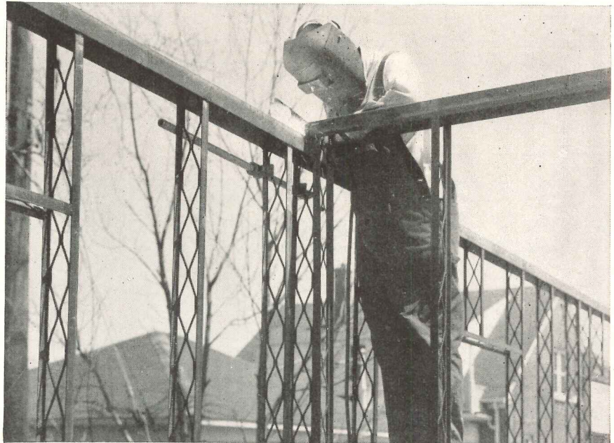
Fig. 1. Arc welding steel panels to form the side walls. Panels are made from 4" Bethlehem expanded steel studs.
