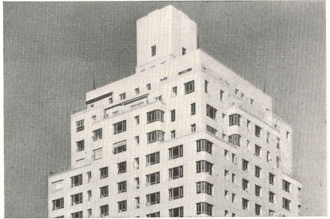
CLASS —One of New York's finest penthouse apartments at 90th Street and Central Park West, where Emery Roth & Sons specified and used the Gold Bond Solid Partition System. Met every exacting requirement. Added 7% rentable space.
