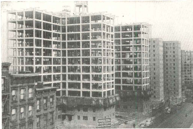
LOW COST —The Gold Bond Solid Partition System, approved by New York City's Housing Authority, helped the successful bidder figure his costs down to a minimum. These are the Amsterdam Houses in New York—1084 apartments.
