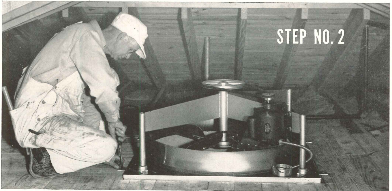
Install the Hunter Package Fan in the Attic ( Fan, shutter and switch in one compact unit )
