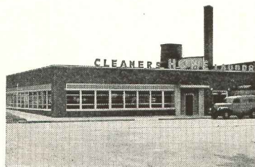
Laundry—Laundry, Bloomington, Indiana. Contractor: Harlos Building Service.
