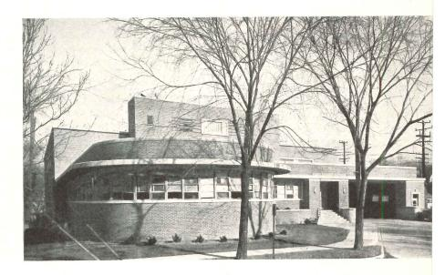
Food stored and processed here is distributed to all kitchens of the University. Merchandise arrives by truck and rail at a receiving dock on the first floor. (Truck entrance can be seen at right; railroad siding is adjacent.) Conveyors take the food from the dock to its storage place on one of the three floors. Orders leave from the shipping dock located in the basement
