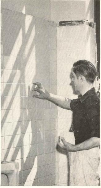
FLOATING TILE on walls with 3M Ceramic Tile Adhesive, Cedar Knolls School. Tile can be set faster; there's less cleanup needed than when mortar is used—further savings which enable the contractor to quote for less.
