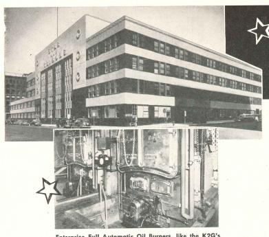
Enterprise Full Automatic Oil Burners, like the K2G's installed in the Star-Tribune building, are widely used to secure the lowest cost heating performance without need of more than occasional inspection.
