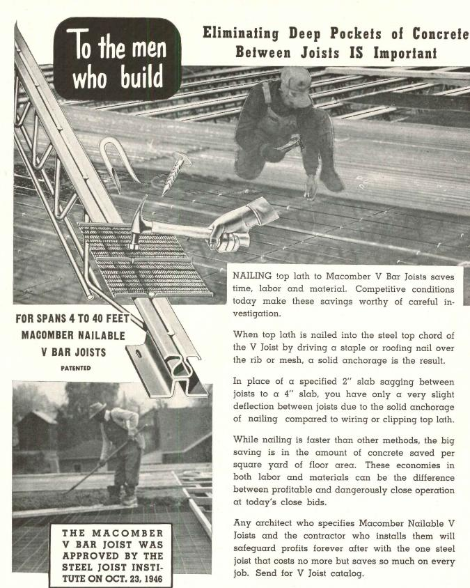
NAILING top lath to Macomber V Bar Joists saves time, labor and material. Competitive conditions
