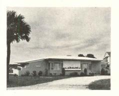
Light-colored marble chips over aluminum foil forms lightweight roofing with good reflective insulation values
