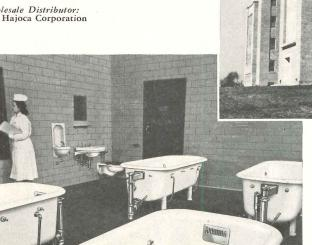
Hydrotherapy treatment room at the Philadelphia State Hospital, showing battery of Prolonged Treatment Baths. The automatically-controlled baths are made of rigid cast iron and finished inside with a heavy coating of acid-resisting enamel. The wall-supported fixtures in background are the Cardic Drinking Fountain, Buena Lavatory and Instanto Water Closet. All are made of genuine vitreous china that is easy to clean, and keep clean.
