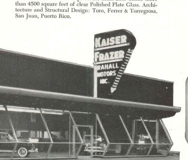
glass applications is its unusual front, glazed with Herculite Tempered Plate Glass. Carrara Structural Glass, Polished Plate Glass, Copper-Back Mirrors and Herculite
