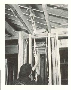
Remote control electrical system uses thin wires (above), has selector switch for 9 outlets (below)
