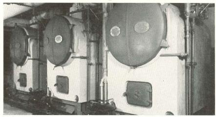
Titusville Boiler Installation of three natural gas fired steel heating boilers in an important southern high school.
