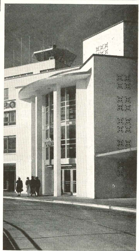
Upper photo shows the terminal building of the Seattle-Tacoma Airport from the ground approach side. Central section is five stories high surmounted by the control tower. In plan the structure is a blunted V, 800 ft. long from end to end of passenger concourses. Total floor area, 243,000 sq. ft. Lower photo shows entrance tower. Grillwork is cast stone. Designed by the staff of the Port of Seattle. Lease and Leigland, Seattle, were the general contractors.
