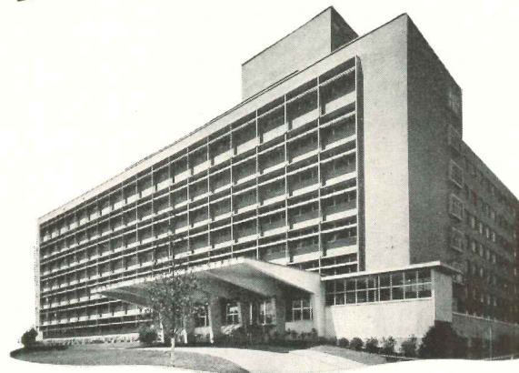
Georgia Baptist Hospital Atlanta, Georgia Architects: Stevens & Wilkinson, Inc.
