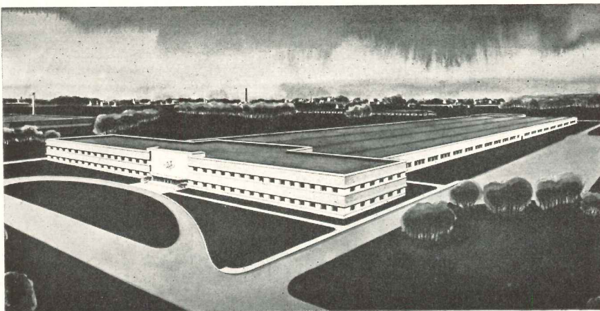
Factory and general office building for Powers Regulator Company at Skokie, Ill.
