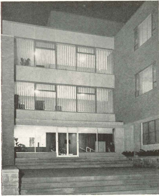
Exterior is brick, backed by masonry blocks on a reinforced concrete frame. Main entrance (above) leads directly to information desk at front of open general office. Main lounge (right) can be extended for special functions by opening up of main and staff dining rooms. Lobby (opposite page) has walnut plywood walls, linoleum floors, acoustic tile ceilings
