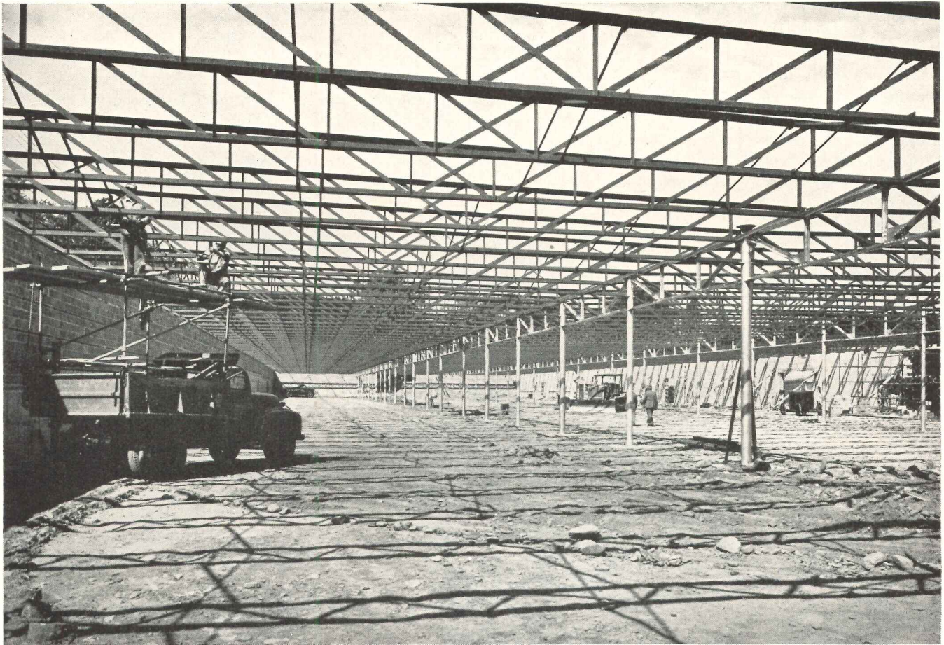
Installation of Bethlehem Longspan Joists in Fernbrook Park Mill (Dallas, Pa.) of Bloomsburg Mills, Inc. Architect: Lacy, Atherton and Davis, Wilkes-Barre, Pa. Contractor: Sordoni Construction Co., Forty Fort, Pa.
