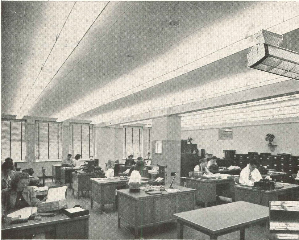
65 footcandles in accounting office from Grenadier lls 6' on centers.
