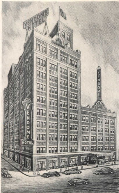
Hotel Vendome, Evansville, Indiana. Architect: Clifford Shopbell, for the original hotel; Fowler & Kargeo, for the new addition. Heating Contractor: H. G. Newman Plumbing Company.
