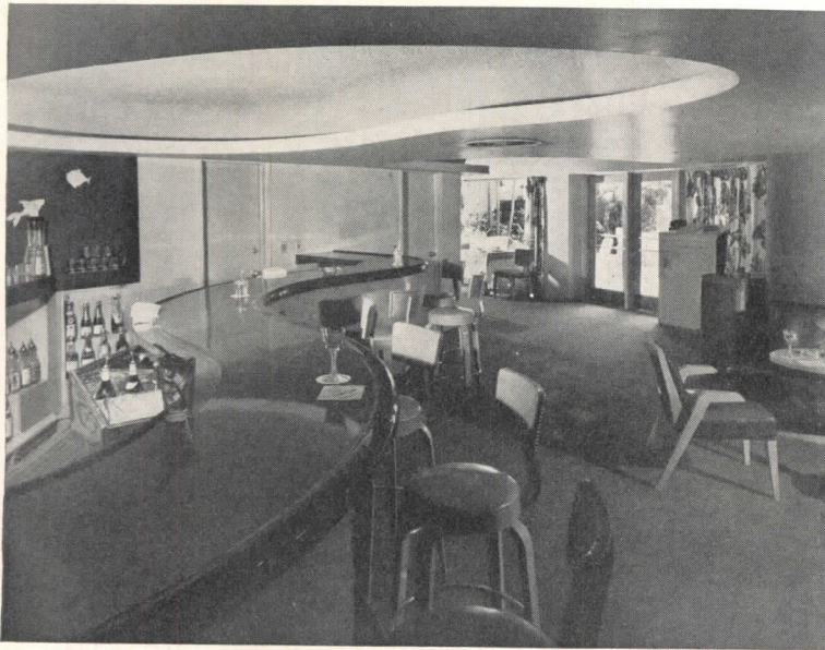
The twin buildings of the hotel proper offer various types of accommodation, including two-bedroom suites with living room and kitchen. Plans above are of second and third floors (lower plan) and fourth and fifth floors (upper plan). Below, left: bar and cocktail lounge, looking toward main dining room. Below, right: a typical bedroom in hotel proper, showing balcony in center rear
