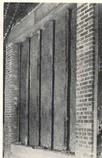
Above: supports for fireproof wall. Below: first exterior coat applied
