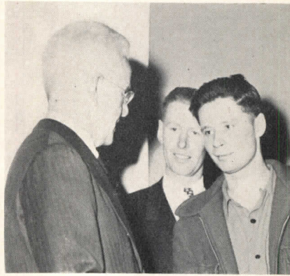
Douglas E. Kertland, Toronto architect, presents Craftmanship Award to Norman Mackay. Center: Bill Nelson of John Nelson & Son Ltd., Toronto plastering firm to which Mr. Mackay is indentured
