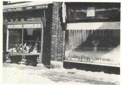
Occupancy of a building determines the amount of water vapor present. Confectioner's store, right, shows high humidity level compared to hardware store, left
