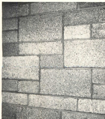
Close-up showing sizes, texture and joint treatment.
