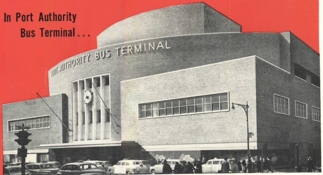
Bus Terminal Building, Port of New York Authority, Turner Construction Co.—Contractor
