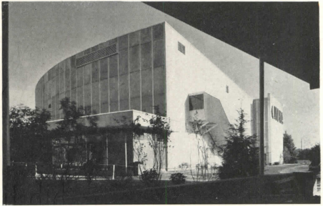
world's largest of steel arched beam construction, biggest in U.S. without interior supports. Its ceiling is suspended on
