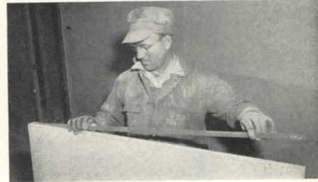
Curtain walls in Leslie R. Porter Co. office (top) are fastened by grooving laminated panel edges (above left) and inserting concealed splines (above right)
