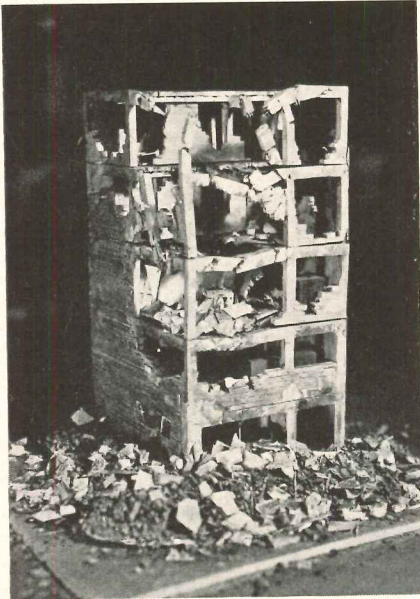
Above: photo of scale model of five-story reinforced concrete office building, hotel or hospital type, typifying bomb damage. Below: "typical" bomb-damaged two-story and basement row house
