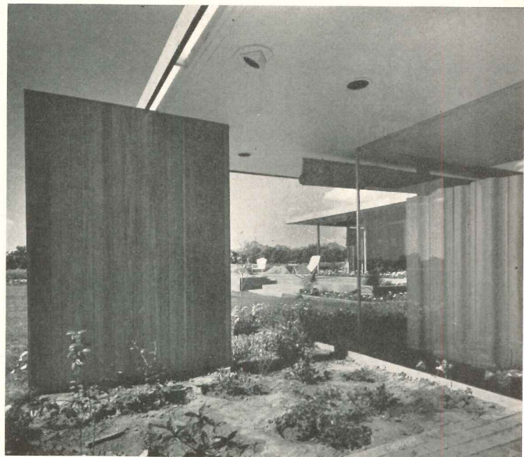
On the plan (opposite page) separate functions are clearly expressed in the four distinct wings. The house is fully air conditioned by means of three separate package units. White gravel roofs, ceiling insulation, and large overhangs reduce the cooling load
