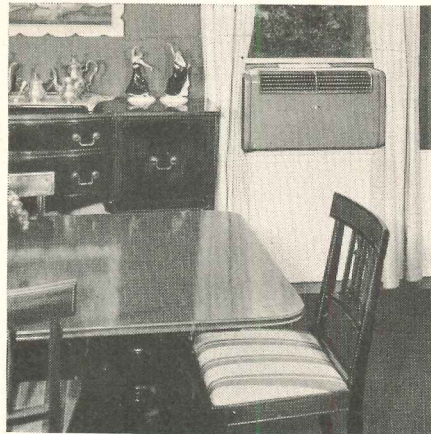
Casement window problem solved with unique use of fixed glass panel.
