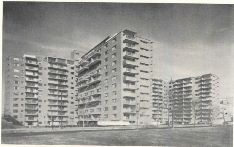
Apartment House, 100 Memorial Drive, Cambridge, Mass.; William Hoskins Brown, Vernon DeMars, Robert Woods Kennedy, Carl Koch, Ralph Rapson, Architects
