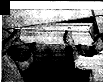
Easy to install. Simply compress the sides of the fixture and insert into grid opening.
