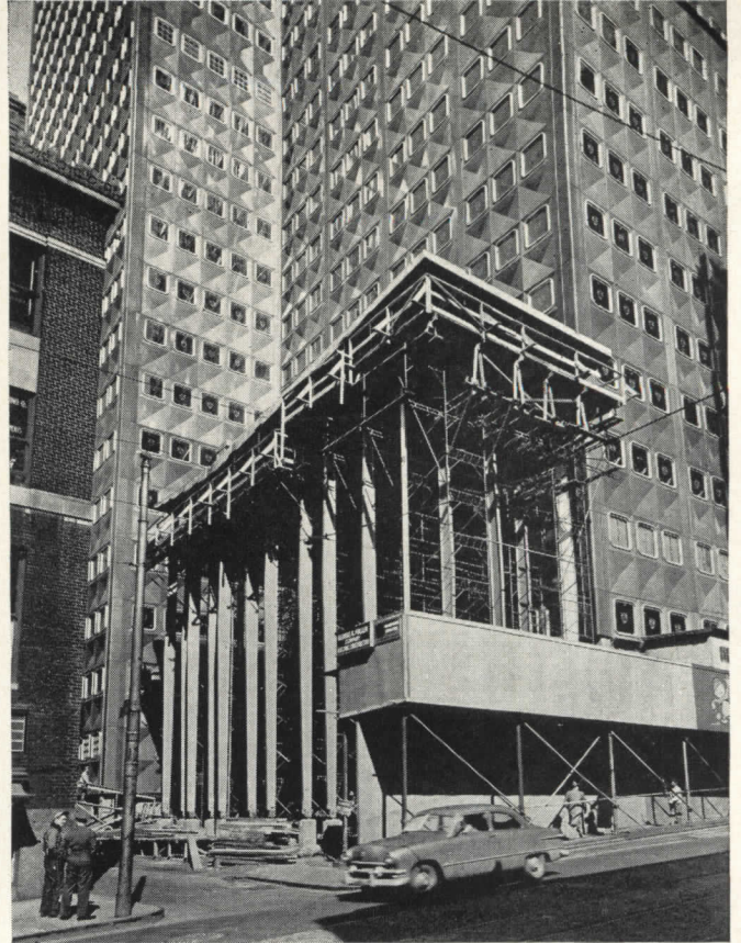
Four and one-half story entrance lobby is suspended from two huge cantilever beams at fifth floor level (above left). The tall aluminum glazed framing members (above) will hold lights of double-glazed plate glass similar to sketch, left
