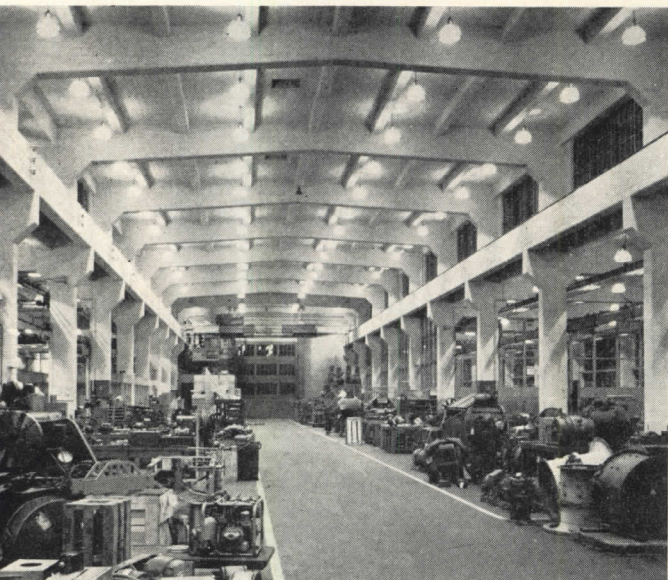
Above: electrical shop, Terminal Island, Calif., is example of concrete rigid frame construction. Right: machine shop, San Pedro, Calif., has thin curtain walls, large areas of corrugated wire glass. Below: warehouse at Naval Supply Depot, Bayonne, N. J., has repetitive roofs of thin shell concrete. Below, right: cold storage building, Oakland, Calif., is of reinforced concrete, has no windows, for easy temperature control
