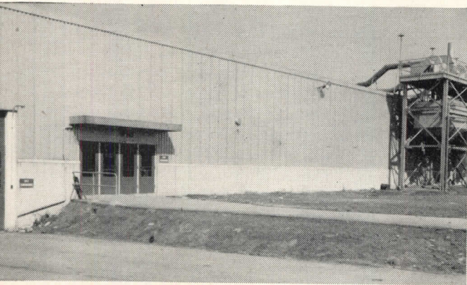
Close-up of the FORMICA plant shows the neat and attractive design formed by continuous Q-Panel fluted texture. Architects have achieved a great variety of design by combining Q-Panels with other materials for decorative effect.
