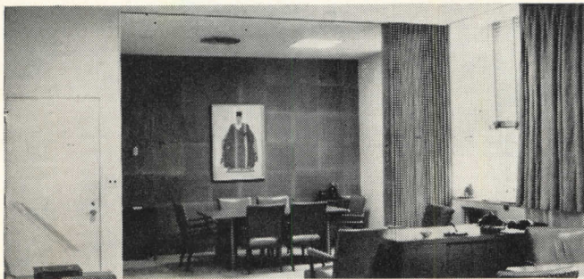
Attractive, modern offices of Henry Sears & Co., New York. Note arrangement of ceiling air diffusers of this central-station air conditioning system.
