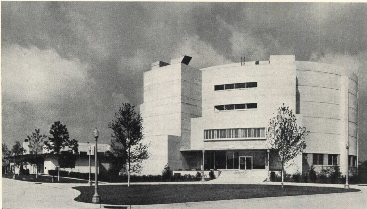
The centrifuge (far right) around which the building was designed, can exert a force equal to 40 times the gravitational pull of the earth on a pilot seated in the gondola (closeup right)
