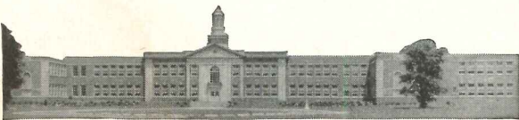
Grade School, Canandaigua, New York Duane Lyman & Associates, architects and engineers, Buffalo; H. J. Bareham & Sons, heating contractors, Rochester
