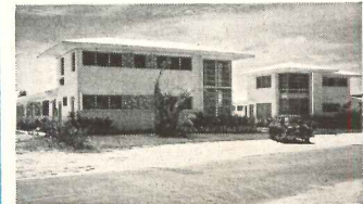
OXFORD APTS. , owner: Jordan Davidson, builder: Jules Block, architect: Don Reiff.
