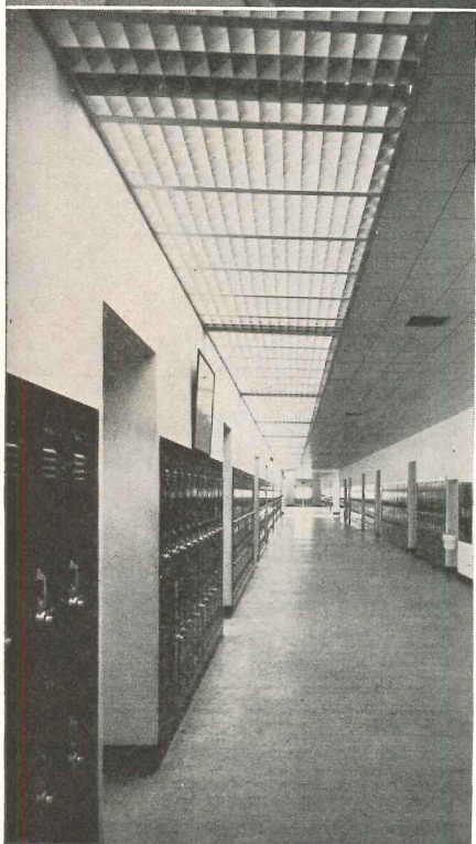
Skylights of new Culver City High School provide daylight illumination in large building.
