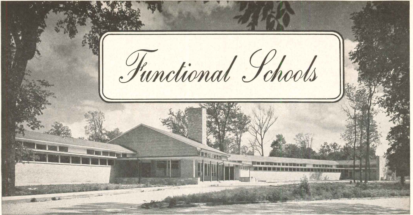
Clyde L. Lyon School, Glenview, Illinois. Walvector in special enclosures along entire walls of windows assures comfort regardless of outside temperatures. Photo by Hedrich-Blessing.
