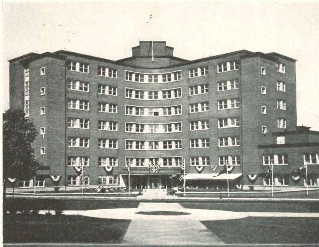
Kitchener-Waterloo Hospital, Kitchener, Ont.; Gowan, Ferguson, Lindsay, Kaminker, Maw, Langley, Keenleyside of Toronto, architects
