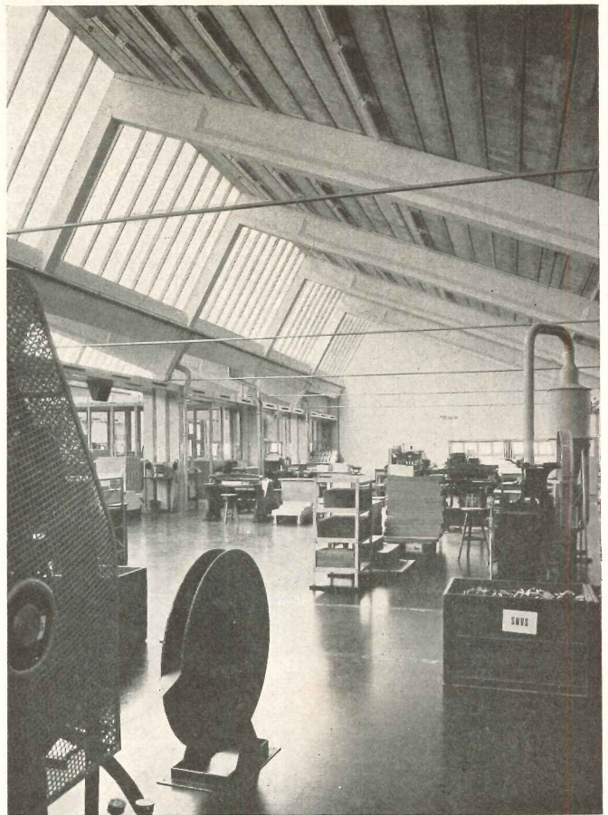
Mullions of the skylight are thin strips of prestressed concrete. Natural light is supplemented by fluorescent lamps mounted on the ceiling. Note how the air conditioning ducts rise up on either side of the column bents and then run horizontally between them
