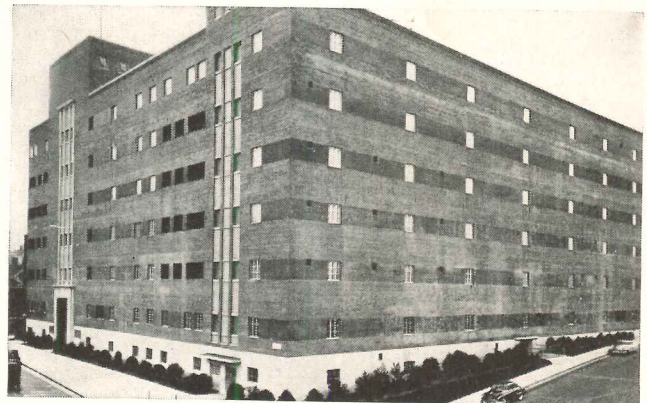
Modern, completely air conditioned cigarette factory of Liggett & Myers Tobacco Company in Durham, N. C.
