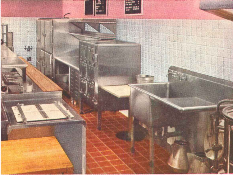
▲ Genuine Clay Tile beautifies the walls of the U. N. cafeteria serving area. At the same time it helps provide the high sanitation standards so necessary in any food service area.
