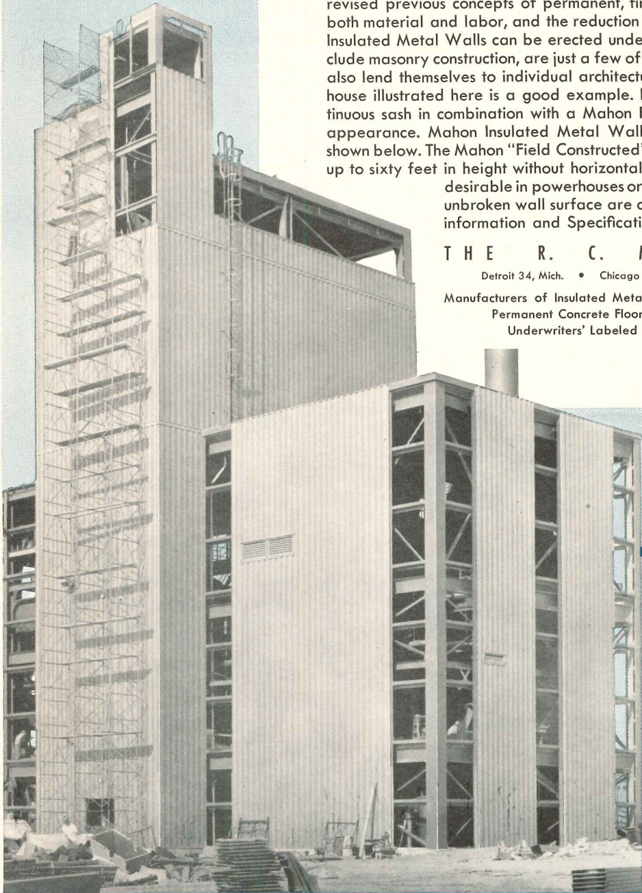
In the Powerhouse above, the Insulated Metal Walls up to the first eave line are constructed without a horizontal joint. Continuous Exterior Wall Plates 56'-10" long were employed in these wall areas.
