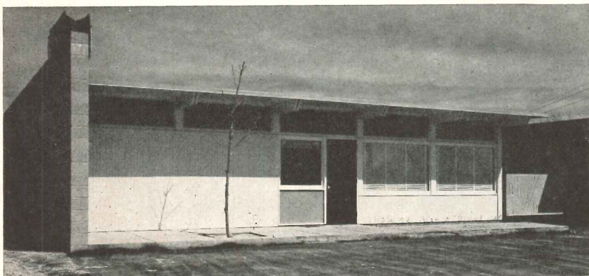
Biggs, Weir & Chandler's building in Jackson, Miss. (below), has white painted siding, bright color accents. Plastic skylights are over central rooms. Drafting tables are separated by tack-board screens in bright primary colors
