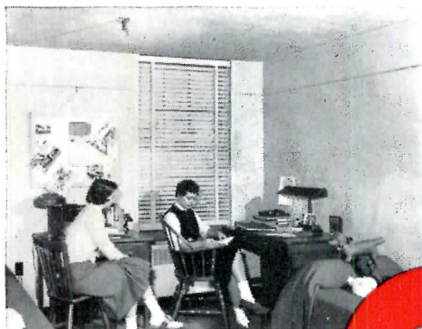
Typical dormitory room, showing regular Grinnell Quartzoid Bulb Sprinkler.
