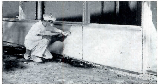
Expansion joint, functional and pleasing, cuts into exterior stucco at 4-ft intervals to interrupt cracks
