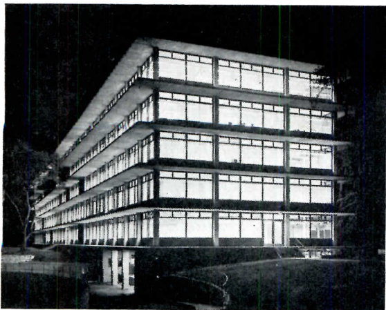
Cantilevered canopies continue around building as expression of flat plate construction, provide sun control, ease building maintenance; structure is dramatically revealed at night. Covered walk (below, right) between lab sciences and auditorium bridges sunken terrace outside cafeteria
