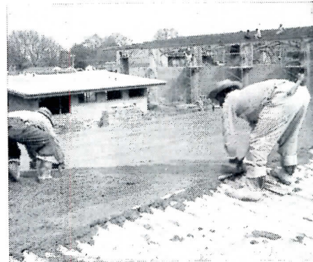
Permanent, Incombustible Roof Deck is provided by cast-in-place slab. When concrete is screeded to depth of 2\frac{1}{2} "-3", load tests show safety factors of 6 to 8 for finished deck.
