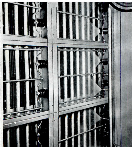
Electronic air cleaner is washed automatically by motorized nozzle. Adhesive is then reapplied
