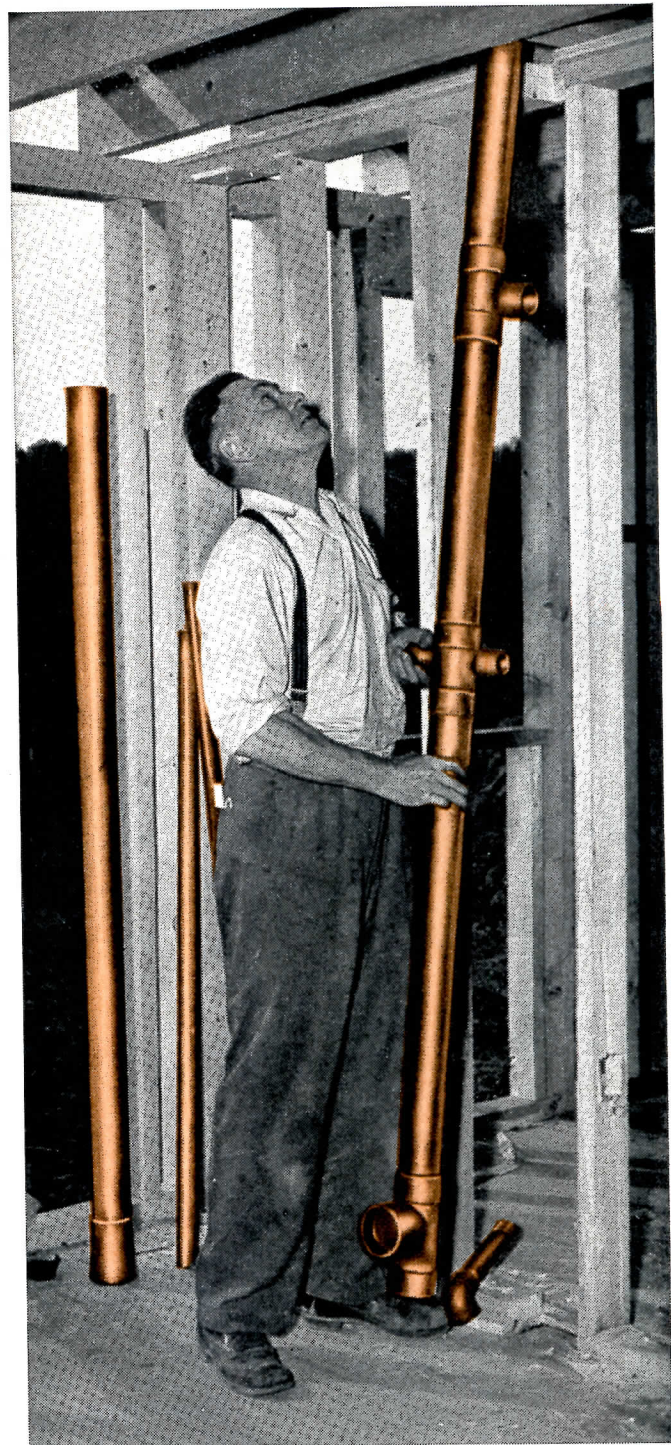
ONE MAN EASILY POSITIONS this 3" prefabricated stack which fits in a standard 4" width partition. Anaconda offers you both Type M Tube and the new lighter-weight Copper Drainage Tube, Type DWV.
