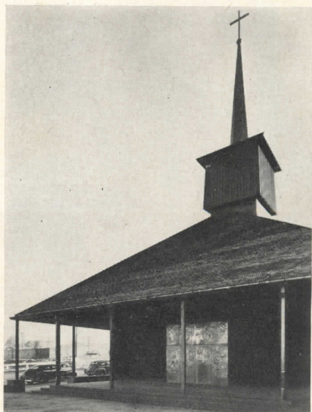
Zion Lutheran Church, Portland, Ore., completed in 1950, Pietro Belluschi, architect
