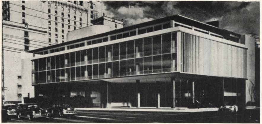
A $2 million library for Vancouver, for which Semmens & Simpson are the architects, will be built on a three ft module, the width of standard bookcases; louvers will be controlled by photoelectric cells
