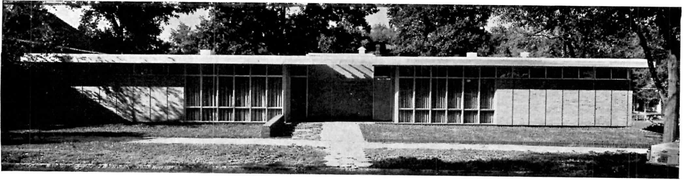
Above: Clinic for Dr. J. L. Wishik and Dr. H. J. Goldstein, Montgomery, Ala.; Donald L. Horton and Martin K. Johnson and Albert L. Williams Jr., Associated Architects. Below: 1. Gretna Methodist Church, Gretna, La.;
