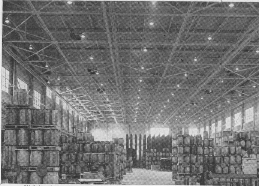
High bay factory lighted by 500-watt incandescent lamps in Abolite GBF Protecto Shields.
