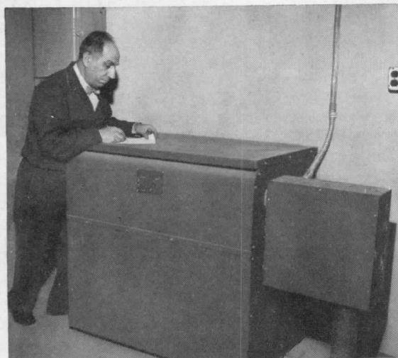
QUIET General Electric dry-type transformers, with low-noise-level characteristics, help improve sleeping comfort for Sheraton guests.
