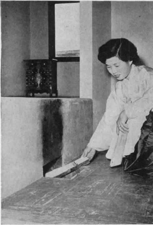
Centuries-old Ondol system uses hot gases from kitchen stove (above left) to heat floors in present-day dwellings.
