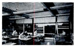
"If fixtures are pendant-mounted, contrast with the ceiling can be reduced, although there may still be light and dark streaks at the spacing commonly used." At John Jay, beamlevel fixtures cast light up on ceiling, down on work surfaces
