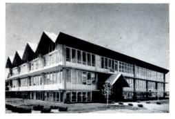
DENVER, COLORADO: Folded plate roof on Denver-Chicago Trucking Company's new office building is of thin-shell concrete. Toll and Milan, architects; Ketchum and Konkel, structural engineers
