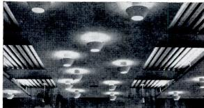
CAFETERIA for Middleville Road High School, Northport, N.Y., features dropped ceiling panels highlighted by a decorative random pattern of gaily colored "spots" adapted from a standard fixture. Fluorescent tubes mounted atop the panel edges supplement the downlighting by casting an even glow over the bright orange-painted cellular decking; above
