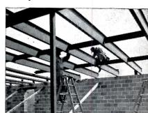
35 tons of 12" JUNIOR BEAMS were used in this Warren Township Elementary School, Indianapolis, Ind. The exposed beams were covered with 3" Tectum insulation, which was topped with roofing. Modular design has windows and columns on 4' centers.
