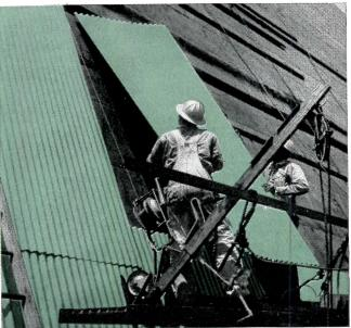
MORE THAN 600,000 lb. of industrial corrugated aluminum sheet was used to roof two huge hangars at Moffett Field. All were treated
