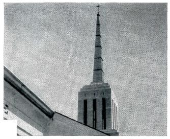
**Plan for strength...** For example, this graceful steeple on St. Dominic's Church, Cincinnati, O. It was built on the ground of rigid, double-locked Monel\* nickel-copper alloy sheeting — then hoisted into place. With strong Monel alloy it will stand up to wind, ice, and snow. It works *with* its masonry setting too — has almost identical expansion.
