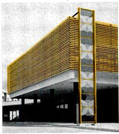
The decorative and functional louvers covering the second floor of this modern structure are extrusions of architectural bronze (see detail at left). The decorative tinted glass panel is framed with Anaconda Red Brass rectangular tube. Architects: Albert C. Martin & Associates, Los Angeles. Fabricator: A. J. Bayer Company, Los Angeles.
