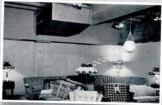
General Electric Celling-Mounted Units at the Dallas Home Furnishings Mart take no floor space —provide Individual temperature control (heat and cool)—are metered for zone control of operating cost.
