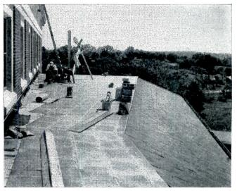
Plan for ease of installation... Monel roofing is easily cut, formed, soldered into place. It's strong, corrosion-resisting... permits the use of lighter, easy-to-handle gauges... takes years of flexing. Roofing contractors don't need any special forming or soldering equipment — and workmen use familiar techniques with Monel roofing.
