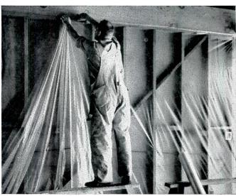
Be Safe: Visqueen film meets Federal Housing Administration Minimum Property and Test Requirements and Federal Spec. UU-P-147B as it pertains to moisture vapor control.
