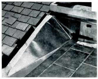
**Plan for durability...** Monel flashings and flat seam work on St. Dominic's will resist pitting, cracking. Monel roofing stands up to corrosive atmospheres, grit, soot. (Today, new crimped forms of Monel roofing sheet also practically eliminate the need for expansion joints — reducing another constant source of trouble.)
