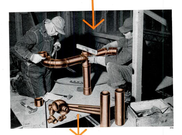
The plumbers here are preparing a Streamline DWV prefabricated assembly for a multiple bath sanitary drainage system. The strong, rigid assembly will be placed into position and completed with a very little additional work.
