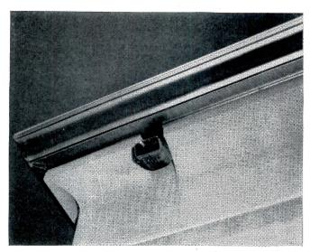
Plan for lasting beauty... This Monel alloy gutter extends the cut stone's classic sweep. Monel roofing weathers to a satin grey that harmonizes with stone. Its corrosion resistance eliminates streaking. Architect — A. V. Walters; General Contractors — Edw. T. Honnert & Sons; Sheet Metal fabricators — Weitkamp and Robinson, Inc., Cincinnati, Ohio.
