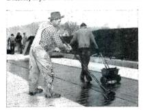
**Semi-mechanical method** is fast for medium or small jobs. Apply ribbons of adhesive with the Lexsuco Spreader, spread ribbons with roller coater and unroll Koroseal into adhesive. Then, imbed insulation into ribbons of adhesive on top of Koroseal. Whether your roofing job is large or small, Lexsuco's engineered application methods cut installation costs.
