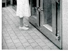
**FOUR-WINDOW** refrigerator front—also stainless steel clad—glazed with three thicknesses of plate glass 1/4" thick. Sturdy hardware is chromium plated heavy cast bronze.
