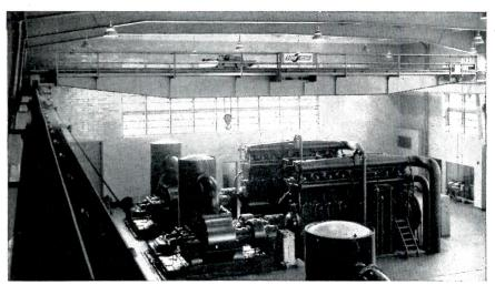
CONCO "CRB" OVERHEAD ELECTRIC TRAVELING CRANE installed in municipal sewage disposal plant.
