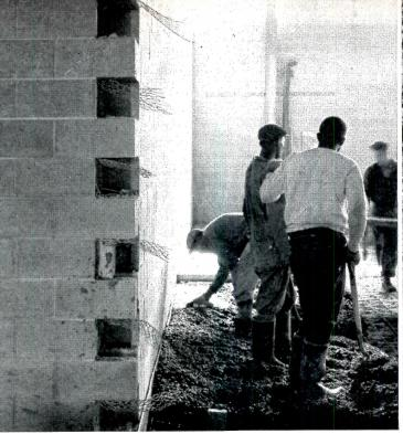
When partition walls are to be built later, Keywall may be cut to extra length to serve as a wall tie. Then Keywall ends may be moved out of the way until needed. Smooth edges of Keywall won't cut or tear hands.
