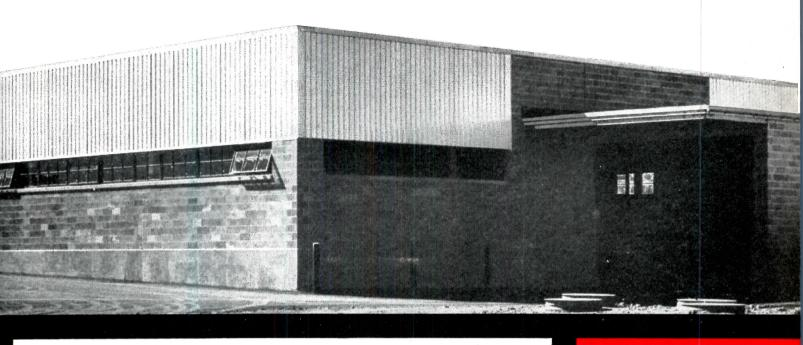
Installed at a labor and materials cost of \$1.50 per square foot, Standard Register's new insulated aluminum sandwich walls were quickly fabricated at the site from a layer of 1"-thick rigid glass fiber insulation—flanked by rugged sheets of lightweight Kaiser Aluminum ribbed and industrial corrugated siding.
