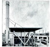
Van-Packer Stack with Hi-Temp Sections handles industrial incinerators with continuous flue gas temperatures of 2000° F.
