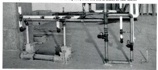
Steel Pipe used for soil, waste and vent lines serving men's toilet room.
