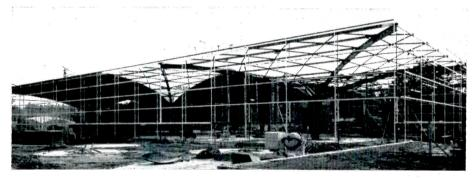
British Industries Pavilion during construction is an airy web of mushroom-shaped supports enclosed in a curtain wall frame of prefabricated timber stiffened by light steel braces
