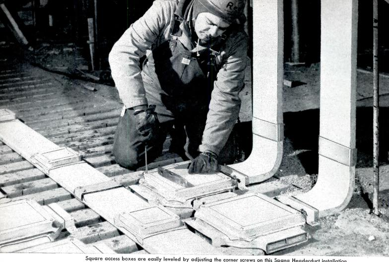
Square access boxes are easily leveled by adjusting the corner screws on this Spang Headerduct installation.
