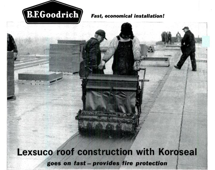
Get a fire-retardant roof fast! Here a Lexsuco mechanical applicator performs three operations on one pass—applies nonflammable Lexsuco Adhesive R907T to underside of Koroseal Vapor Barrier, lays and secures the Koroseal to the deck, and puts ribbons
