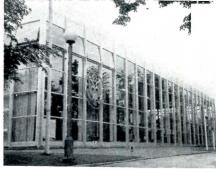
Fabricated in Italy, the large building is steel with three walls of glass supported by vertical aluminum frame members; the other wall is of asbestos paneling. Unobstructed exhibit space is achieved by means of welded tubular steel trusses fastened to round steel columns on the perimeter. The concrete floor slab is laid over electrical ducts. The building is 170 ft long, 95 ft wide, and 32 ft high.
