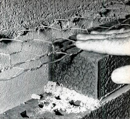
Note how readily Keywall adjusts to variation in brick and masonry courses. Here it serves as tie between brick and block.
