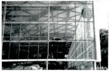
Quickly-erected frame for glazed curtain wall is of low cost, glue-laminated timber
