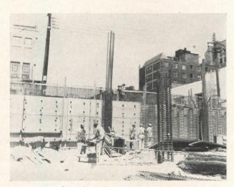
This photo shows first and second story column verticals extending above the basement floor after having been butt-welded to the dowels in caisson tops. Bars are No. 18S high strength types furnished by Republic Steel.
