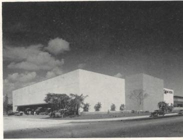
The structure of the building is reinforced concrete frame throughout except for the composing room area which has an 85-ft trussed steel roof for maximum flexibility of equipment layout. Office exteriors are finished with anodized aluminum curtain walls; production area exterior has precast concrete panels (with exposed aggregate), except large enclosed press area which is of brick for contrast
