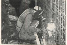
Inner and outer mats are welded at laps (above), joined by brazed leads. Leads also join mats to structural members (below)
