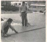
BETOCEL mix has consistency of thick malted milk. On installation, it sets up to form a unique cellular structure providing all these advantages:
