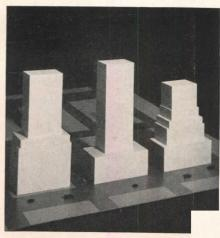
Left to right: 1. Open area at ground level permitting higher rise before initial setback, with tower above; 2. Maximum bulk up to required initial setback, with tower above; 3. Maximum bulk using proposed standard envelope, with no bonuses
