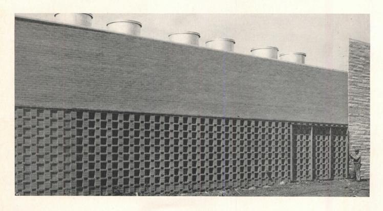
When it's ten below zero in Chicago, the heat pump system in a new 220,-000 sq ft suburban factory will produce a total of  $5\frac{1}{2}$  million Btu per hr—enough to heat 300 average-sized houses. According to industry sources, this is the largest air source heat pump ever installed. Six big fans pull in a total of 250,000 cu ft per minute of outside air across refrigerant coils, extracting heat and in the process cooling the outside air down from -10 F to -20 F.
