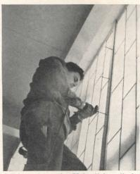
Joining system for Kalwall installation is simple. Inner and outer battens, are coated with a sealing material—then fastened to each other with long screws. Battens seal panels to each other—play no structural role.
