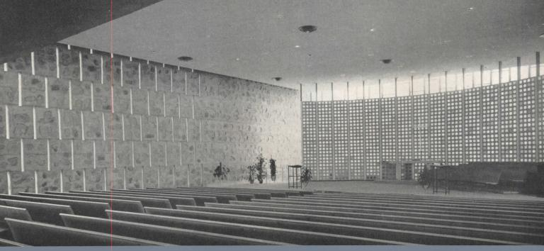
Roof is steel deck on long span joists. Ground slopes downward sharply where stairs lead to a general purpose and dining room in the basement. Glazing extends from basement floor to fellowship hall ceiling
