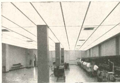
Installation of Contrex Soundsheet — Operating Room, Forest Hills Telephone Building, New York Telephone Company.
