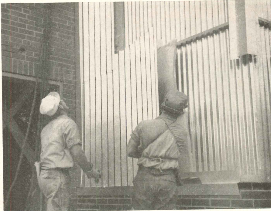
Walworth Company, Glenshaw, Pa. Designed and constructed by: The Rust Engineering Co., Pittsburgh, Pa.
