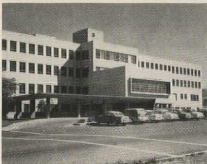
General Hospital, Ventura County, California . . . 400 beds. A Cat D397 Electric Set supplies standby power for operating room, delivery room, emergency room, iron lungs, X-ray machines, laboratories, heating, air conditioning, kitchens, refrigerators. Power is delivered to several buildings.
