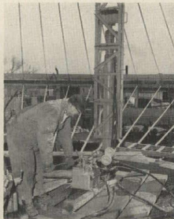
Left: tightening up the bolts on the top tension ring after the cables had been strung. Center: to get initial prestressing of cables, the two steel tension rings were jacked
