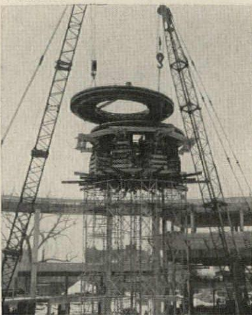
After the inner steel tension rings were fabricated, cranes hoisted them to a central tower topped with wood blocking.
