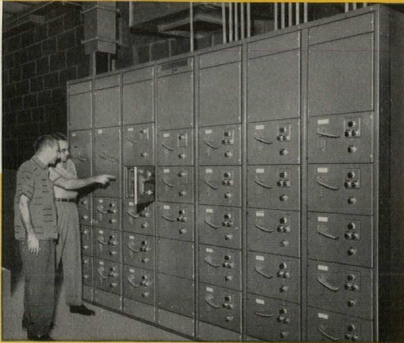
This SQUARE D CONTROL CENTER centralizes all motor control for units which air-condition the lobby, foyer entrances, offices, dining rooms, cocktail lounge, night club and casino. Pumps for chilled water system and swimming pool are also controlled from this center. SQUARE D totally enclosed FEED-IN DUCT brings power from substation.
