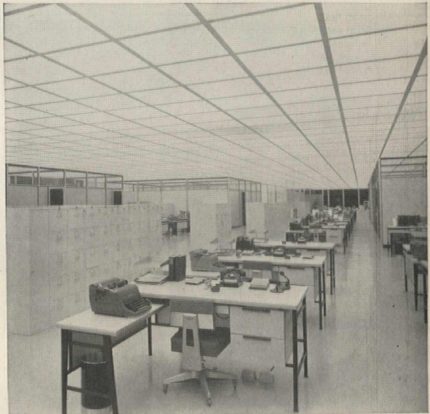
Large office areas are as effectively illuminated as small areas with a high degree of visual comfort assured. In this special Curtis grid installation, aluminum materials were used throughout. Maintenance features of the system include ease of relamping, ready access to wiring, simple replacement of ballasts.
