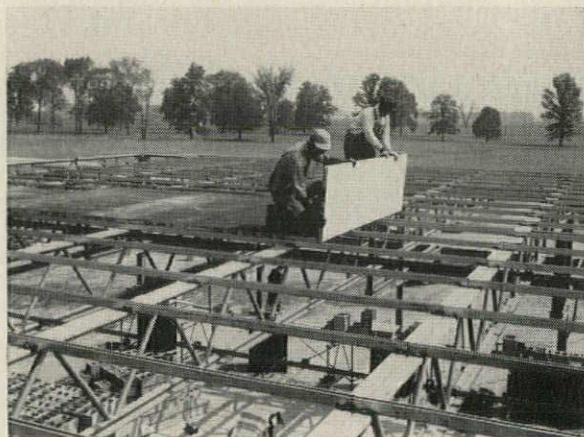
The new Tectum roof deck assembly offers many advantages for commercial, industrial and educational buildings.
