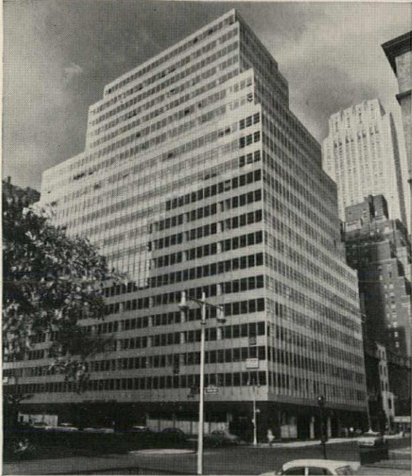
NEW YORK CITY: LUPTON supplied and installed Type "H" fabricated aluminum curtain-walls for this building at 300 Park Avenue. Mullions are aluminum tube with expansion joints at alternate floors. Non-insulated spandrels of opaque structural glass were used. Architect: Emery Roth & Sons.
