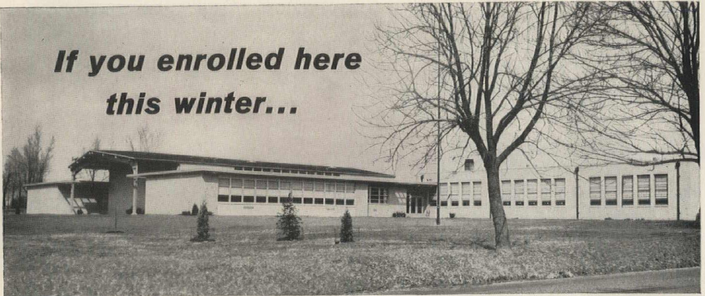
College Corner School, Anderson, Indiana
