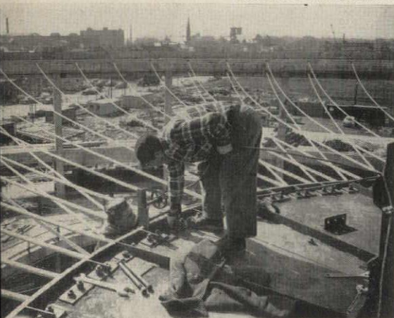
Left: tightening up the bolts on the top tension ring after the cables had been strung. Center: to get initial prestressing of cables, the two steel tension rings were jacked
