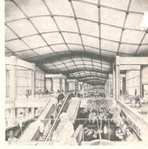
Philip Johnson, Philip Johnson Associates: undulating roof is made of grid of steel pipes which support precast concrete roof planks. Structure front has lower stone facing, upper decorative grille
