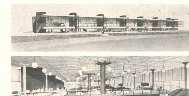
Morris Ketchum, Jr., Ketchum and Sharp: stairwells divide building into 7 glass-walled sections. Columns support concrete roof with radiating roof structure
