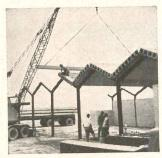
New 8" x 16" Hi-Stress units are fully prestressed slabs ( $f_{\rm si}$  175,000 psi) cast in steel forms, with stress-relieved strands tensioned before concrete is poured. Appearance is similar to standard Flexicore slabs which use pretensioned intermediate grade steel bars.
