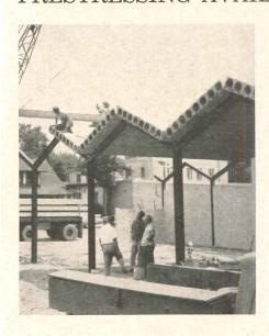
Flexicore precast concrete floor and roof slabs are now available as prestressed units which give longer clear spans and greater load carrying capacities than the company's standard units. High-tensile wire strands are tensioned before the concrete is cast in steel forms.
