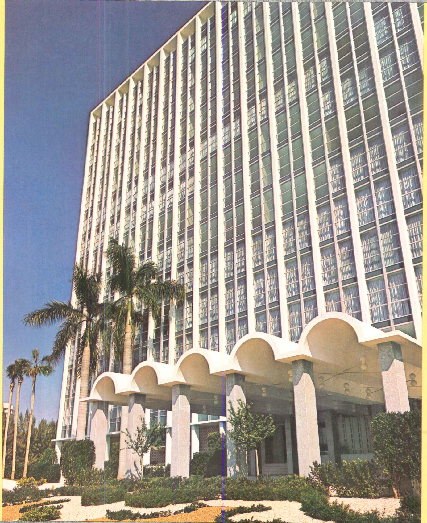
Crystal House apartment building, Miami Beach, Florida Architect: Morris Lapidus, Harle & Liebman, New York-Miami-Washington, D. C. Contractor: Robert L. Turchin, Inc., Miami Beach, Fla.
