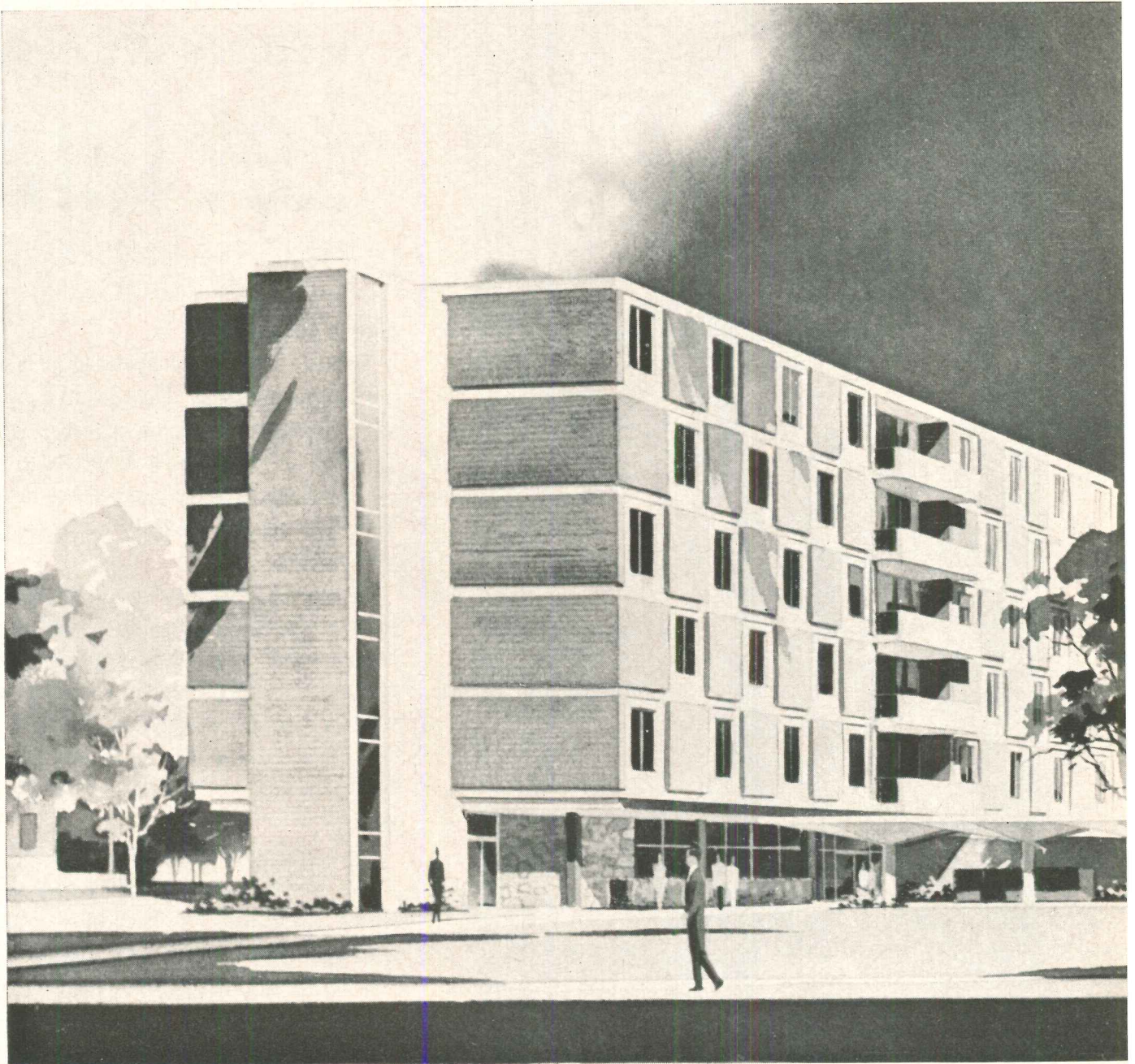
AMERICAN LUTHERAN RETIREMENT HOME , Fargo, North Dakota—the state's first pre-stressed lift-slab building. Each of six post-tensioned slabs measures 103' x 47'. Maximum column spacing—24' x 15'11". Architect: Foss & Co., Fargo Moorhead. General Contractor: J. E. Kreig & Sons, Inc., Fargo. Consulting Engineer: Kolbjorn Saether & Assoc., Chicago. Lifting Contractor: Northwest Lift Slab Co., Portland, Oregon.
