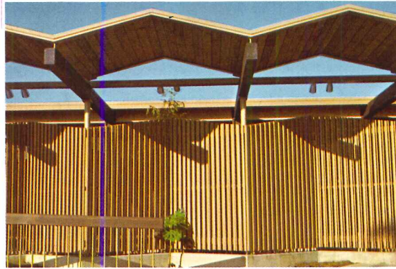
Simple application technique of 1" x 2" Western Red Cedar produces dramatic, but practical result for privacy screen.
