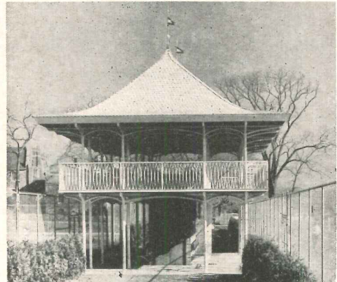
Tennis Pavilion at Princeton University Princeton, New Jersey Architects: Ballard, Todd and Snibbe Structural Engineer: Peter W. Bruder General Contractor: Matthews Const. Co.
