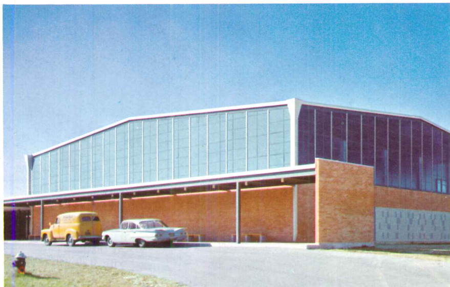
Coolite, heat absorbing glass controls light and temperatures in Parkway Consolidated School, St. Louis, Missouri. Architect: Schwarz & Van Hoefen, St. Louis. General Contractor: Swan Construction Company.
