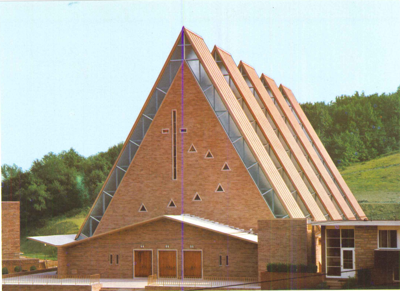
1/4" Hammered Misco glass glazed in roof of St. Sebastian's Catholic Church. Architects: Gerard & McDonald—M. W. Stuhldreher Assoc., Pittsburgh. Glazing Contractor: Golomb Paint and Glass Company, Pittsburgh. Photos of St. Sebastian's Catholic Church courtesy of Aluminum Company of America.
