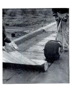
A new idea in built-up roofing consists of a 3-ft-wide mastic tape which is applied cold to flat or sloping surfaces. Under development at Koppers laboratories for more than four years, commercial production is expected later this year.
