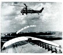
day. The roof, 150 ft above ground, has a 2- by 6-in. tongue and groove southern pine decking furnished by the Forest Products Div. of Olin Mathieson. Arches and purlins were pressure treated. *Unit Structures, Inc.*, Pestigo, Wis.
