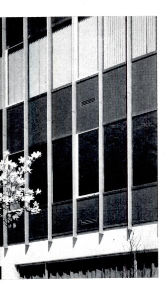
The structure of the 777 Summer Street building is steel frame with bar joist floor and roof construction. Floor and roof slabs are poured concrete on metal decking. Interior partitions are plastered concrete block, solid gypsum board or metal stud and gypsum board, painted or with vinyl wall covering. Flooring is terrazzo on the ground floor, asphalt tile on the stories above. Exposed grid, mineral acoustical tile is used throughout the building.
