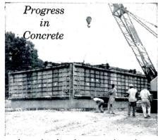
A complete form for concrete house being lifted by crane. The unit, of Symons Forms, has 5,000 square feet of surface.
