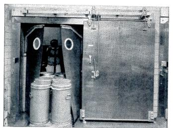
SAVES REFRIGERATION. Jamison Manual Horizontal Sliding Door in combination with self-closing Flexidor®.
