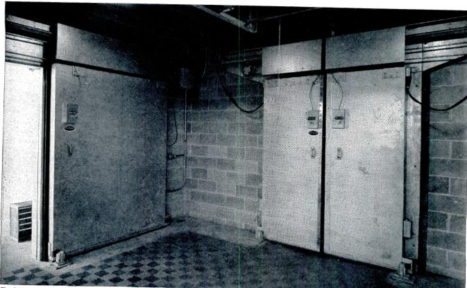
FAST OPENING AND CLOSING. Jamison Electroglide® Power Doors speed traffic to loading dock—single leaf cooler door, left, and bi-parting freezer door, right.
