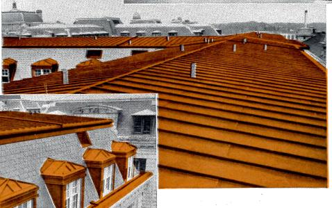
**CLOSE-UP** of dormers, deck molding, vents and gutter of Revere Sheet Copper. Outside section of gutter is lead coated copper.
