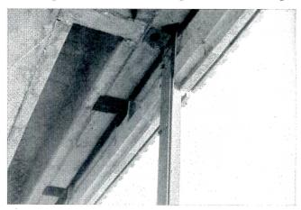
irons—here pictured—stud bolts near the bottom of the panels were secured to stud bolts in sill bottoms. Installation thus was fast, firm, and effective.
