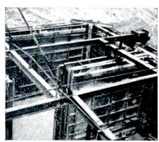
Lifting pads are welded to 8" 1-beams that tie assembly together. Tension rods strengthen unit and keep it square.
