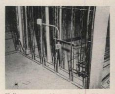
Hollow core provides space for wiring
