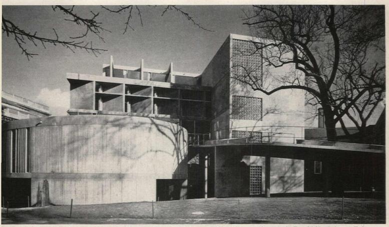
Carpenter Center from Quincy Street: each floor has indoor, outdoor terraces. Concrete baffles shield window wall from sun
