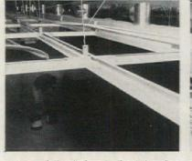
A specially designed direct hanging clip spaced 4' 6" on center supports the suspension system, including light fixtures.
