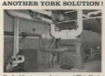
Cool with steam or hot water ! This York absorption type unit provides economical water chilling for air conditioning wherever there is a source of low-cost steam or hot water.
