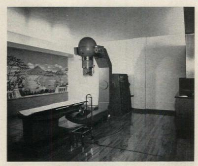
The cobalt-60 unit is located in a room on ground floor, specially arranged and protected to lessen the hazards of radiation scatter. Walls are plaster; floors, vinyl tile
