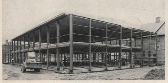
Lightweight partitions avoided the need for intermediate support of precast slabs
