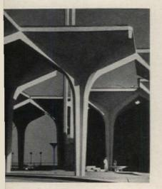
The simple structural system—based on a 40-foot module—consists of a series of spreading columns made by tying together four precast, L-shaped bents; plus thin roof slab elements that serve to lock the entire frame together. The precasting operation was carried on at the site, and had to take place at night, due to rapid evaporation and the extreme daytime heat, often 130.
