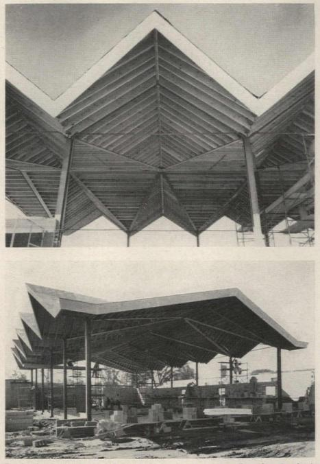
Tension band of high-strength steel bars in effect "prestresses" wood roof to let it float atop the steel columns. Walls have large expanses of glass to give spacious feeling. Project includes sanctuary plus connecting classroom building. Architect in charge of design was John Evans; engineer was Alex M. Cytrynowicz
