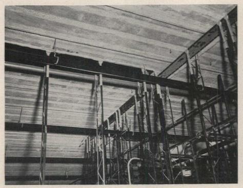
Metal lath partitions are isolated from ceiling deck by a 1/2-in. fiber glass pad
