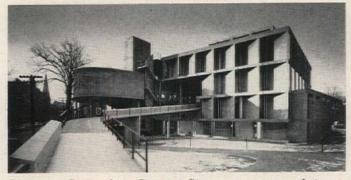
Carpenter Center from Prescott Street: ramp passes between glass-walled workshops and terraces at third floor level. Columns 22 feet high support overhanging third floor lobe
