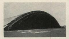
which are roof, ceiling, structural frame and shell of the building. Steel struts separate and connect the two skins. Behlen Mfg. Co., P.O. Box 287, Columbus, Neb.
