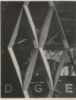
Lattice-like truss wall of I.B.M. Building, Pittsburgh, is sheathed in textured stainless
