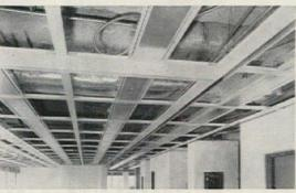
Ceiling construction is made up of 4' 6" x 4' 6" module. Main runner pans 3t/2'' x 13' 6" length, cross pans 3t/2'' x 4' 2t/2'' lengths.\* (Partition ceiling channels are also attached to this assembly).
