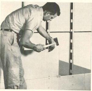
Gypsum lath being attached to Gold Bond nailable steel stud.
