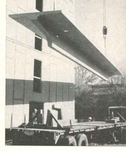
Prestressed channels span 36 ft; are supported by inverted T's set n columns. Pipes and straps temporarily brace columns
