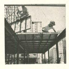
Symons Slab Shore System uses Symons standard Steel-Ply Forms, normally used for vertical wall forming, for all decking requirements. Material adaptability, ease of assembly, speed of erection and stripping are among its advantages over conventional flat slab forming.
