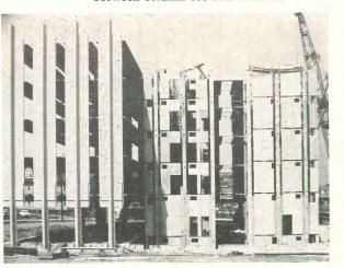
Precast walls and columns become monolithic by casting in place horizontal and vertical joints
