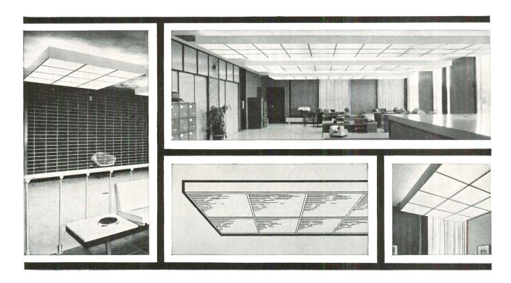
Here's a refreshing way for lighting specifiers to depart from conventional row-type fluorescent lighting installations. The Panelaire series utilizes large floating panels of light to achieve high levels of illumination while maintaining effective control of direct and reflected glare.
