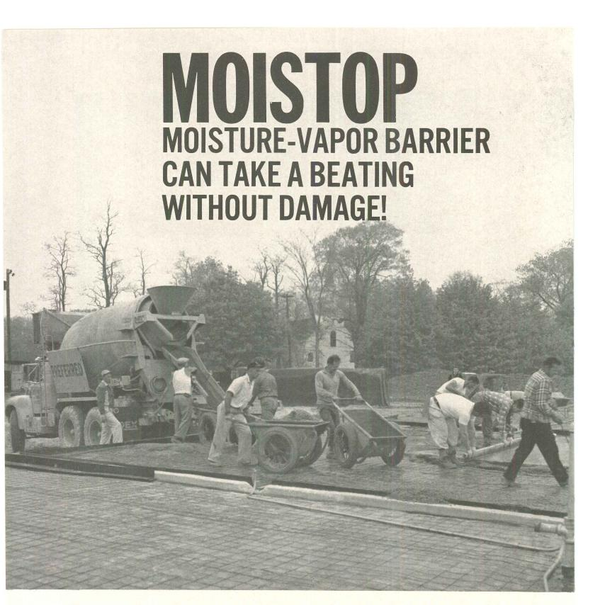
This is the kind of rough treatment that a lot of vapor barriers, including 6 mil polyethylene, just can't take! Rips and punctures will allow moisture to get through. But superstrength MOISTOP won't let this happen! Moistop is a combination of tough, reinforced, waterproof Sisalkraft plus polyethylene . . . this combination is far tougher than polyethylene by itself.
