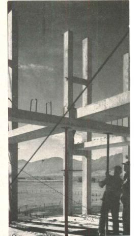
Cast-in-place concrete ties the whole structure together for continuity
