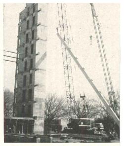
Cranes hoist 86-ft-long precast column; i will be braced against elevator tower at lef
