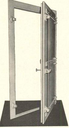
Fallout shelter: This Overly blast-resistant and radiation shielding door was installed to protect a special fallout shelter at the Ohio Power Company, Canton, O. Constructed of heavy gage metal, the door contains a lead core that acts as a radiation shield.
