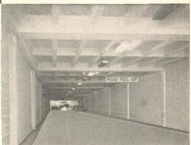
Interior view shows double tee and concrete masonry construction.
