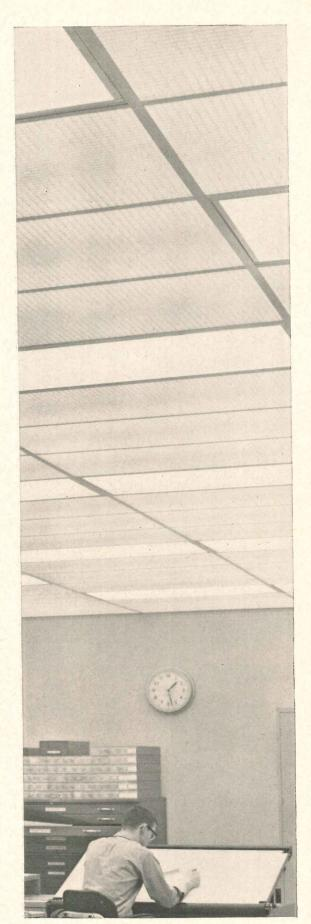
Unusual but highly effective is this installation of Sylvania's Sylva-Flo (air-handling) Troffers in a Sylva-Cell (illuminated) ceiling. This application provides the combined comfort of high-footcandle lighting and outstanding air conditioning performance.
