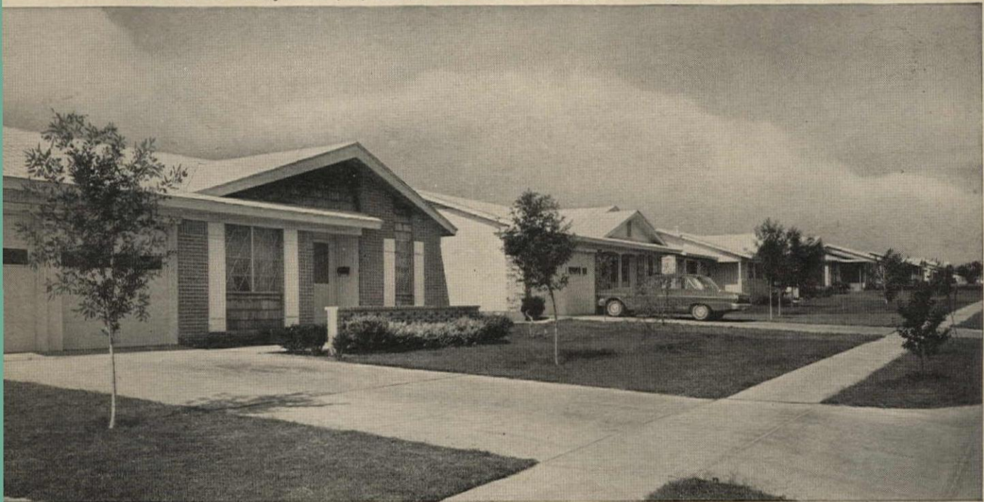
Builder Fred Peek specified York Central Air Conditioning for these fine homes in Richardson, Texas. Architect is David M. Sweeney.
