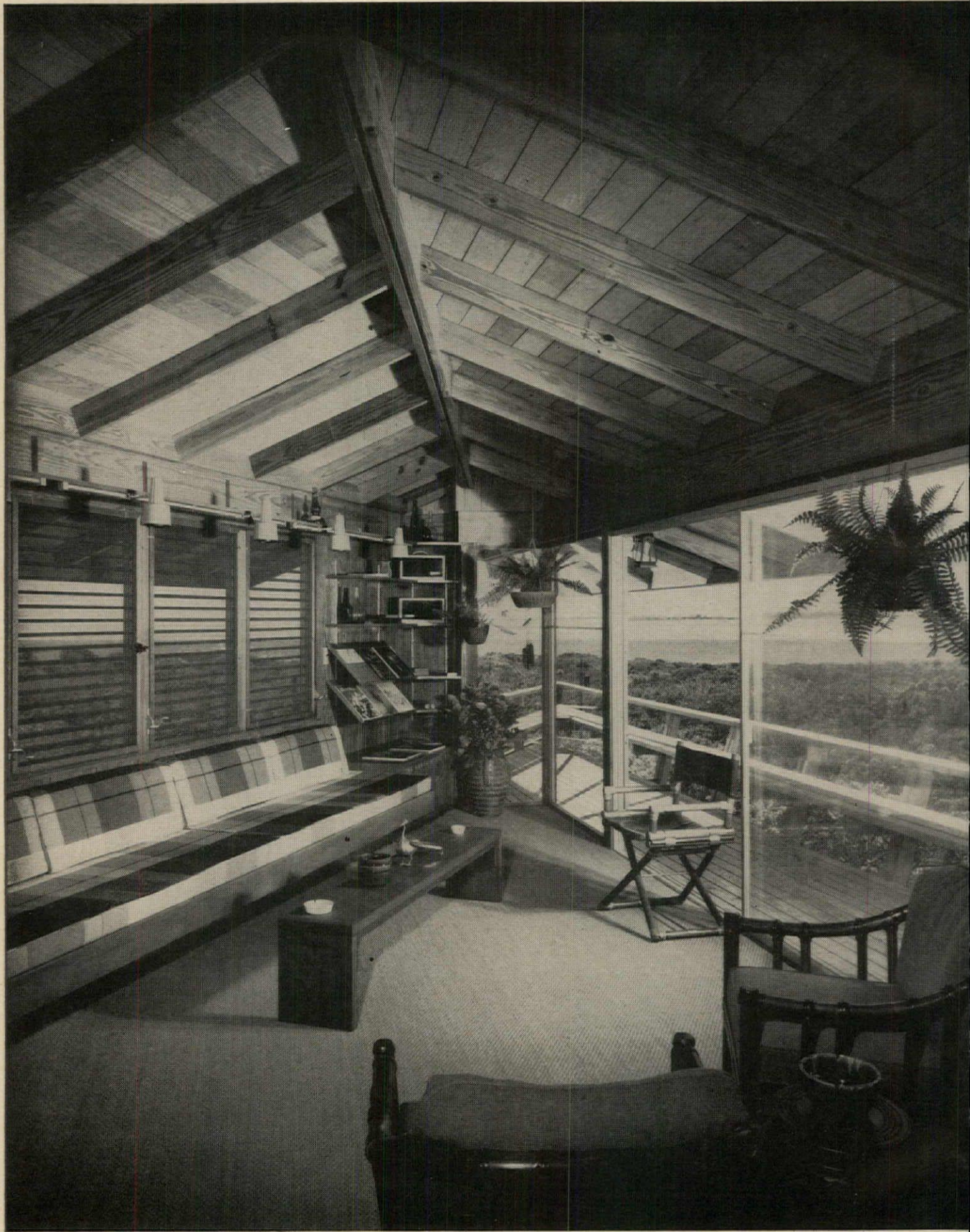
A vacation hideaway in the Bahamas uses wood converging beams and rough-sawn ceiling to work wonders in its very livable, triangular living room. Note the complementing wood built-ins designed by The Richard Plumer Company, Miami, for this Frazer Hog Cay cottage.
