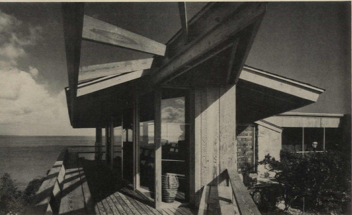
Spectacular exposure on every side makes the Frazer Hog Cay cottage sure of its site. Wood decking, railing, and unique roof supports show wood's way to resist occasional high wind storms, yet maintain a serene retreat from the busyness of daily living. Architect: Peter Jefferson.
