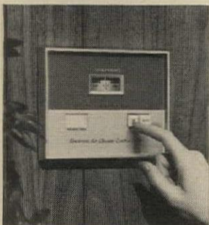
Handsome panel in living area shows cleaner efficiency. Signals when unit needs cleaning.
