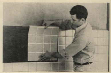
Test applications of American Olean's new *Master-Set* glazed tile sheets indicate a substantial saving in installation time, when compared with individual tile setting. Tests carried out on a 9- by 18-ft wall showed that a team using the new *Master-Set* mounted tiles could complete the job in about half the time it took them to surface the wall setting each tile individually.
