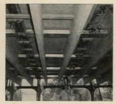
Note ductwork passing through web of tees. This method used to conserve overhead space.
