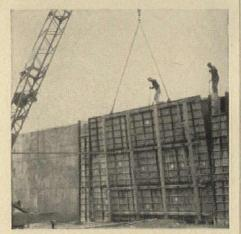
Concrete subcontractor, Alsan Masons, Inc., North Brunswick, New Jersey, averaged 56 lineal feet of 18 ft. high, 12 inch thick basement walls (including two projecting concrete pilasters) each working day. The job: A two-story and basement department store (260 by 560 ft.) in Woodbridge, New Jersey, shopping center.
