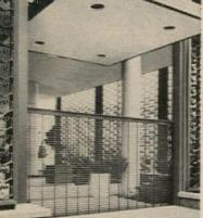
Two of several Cookson Grilles installed in the modern new Bay View Federal Savings and Loan Association building. San Francisco. Top view shows exterior Side-Coiling Grille in unusual curved track design. Inset shows one of the upwardacting Cookson Grilles mounted in the floor. All are power operated. Architect: Fischer, Miyamoto & Bassett. Contractor: Barrett Construction Company.
