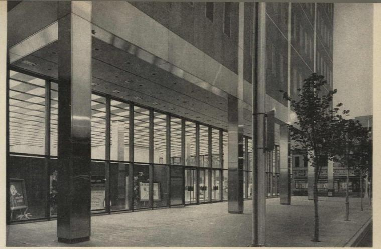
Set back from the building line and shaded from morning sun by the building overhang, the entrance is the midpoint of a glass wall that encloses the ground floor on two sides and acts as a display case for the company's service and sales. Snow melting equipment, using 27 watts per square foot, is installed in the sidewalk around the building; infrared lamps in the soffit of the overhang direct heat down in from the show windows. The checkerboard
