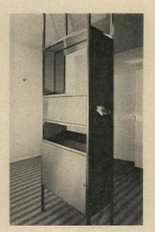
In records department, luminous ceiling provides high lighting level. The free-standing towel holder used in toilet rooms throughout building, contains two towel dispensers, two dryers, two mirrors and one towel disposal in cabinet 1 by 3 feet. Drinking fountain is of cast brass, chrome plated and dulled. Fountain and towel holder where specially designed for the building
