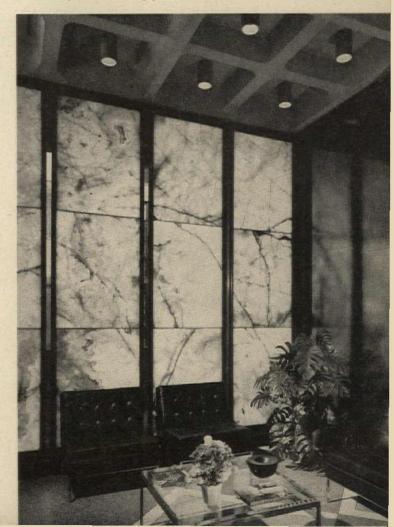
First floor walls consist of translucent glass, clear or obscure glass and translucent onyx panels which can be seen in photographs at right. The onyx panels are separated by clear glass slits. Ceiling waffle slab is left exposed. Other exposed concrete surfaces are sand blasted
