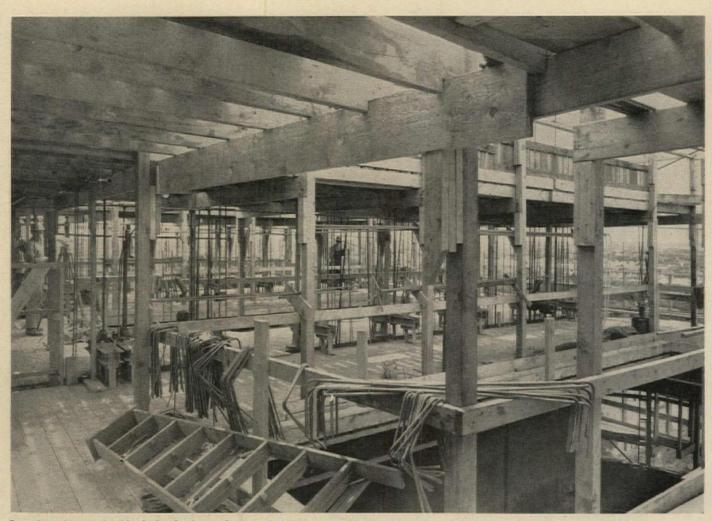
Interior view of double-deck platform shows reinforcement in foreground; row of jacks can be seen in center of photo
