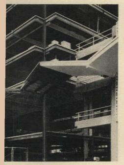
700 tons of Bethlehem steel, most of it V50, was fabricated and erected by Trojan Steel Corporation, Columbia, S.C.
