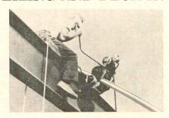
is designed to slide and interlock with the leg of the adjoining section to provide a complete roof assembly. The material is cut to the specified length in the plant and is shipped in straight sections to the site where it is curved to the radius of the arch. A man sitting on the main arch sup-
