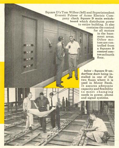
Electricity contributes substantially to the over-all efficiency, convenience, safety and comfort of this most modern banking facility. There are 60 miles of control wiring alone. The monthly power requirement would supply 800 average homes.
