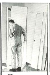
Side panels insert into front frame; edges are routed to fit channels. Back panels (if used) slide into side panel grooves. Panels bolt to shelf support angle.
