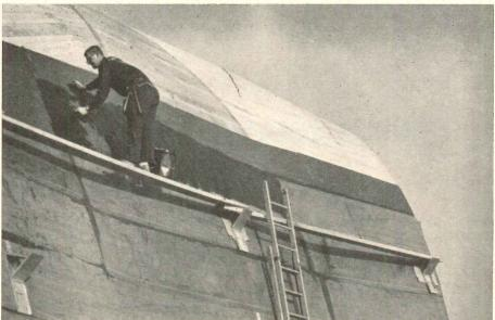
Substrate irregularities should be minimized since they may "telegraph" through roofing. Here insulation board was nailed to wood deck; adhesive is troweled on
