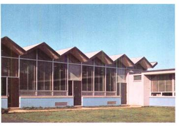
Hollow structural sections are used as compression members in folded-plate, steel-deck roof. Sections transfer shear to the columns. They also act as exposed backup for the windows: Architect: Nicholas G. Eckert, New Brunswick, N.J. Consulting Structural Engineers for all structures shown on these pages: Schwartz & Senes, Englewood, N.J.
