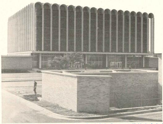
Ceramic Cooling Tower built in August, 1961, at Texas Technological College, Lubbock, Texas. Two Cells; 3,520 GPM; Specifications °F: 100-85-74. Architects: Davis, Foster, Thorpe and Associates, Inc., Architects and Engineers, El Paso, Texas; Consulting Engineers: Zumwalt & Vinther, Engineers, Dallas, Texas.
