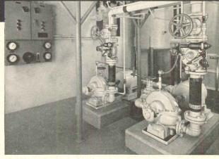
The pump room of the Belle Plaza illustrates the compactness of a Type II Uni-Pressure System. This equipment is designed to provide a minimum of 150 GPM and a system pressure of 83 psi.
