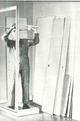
U-shaped shelf support angle, with hang rod attached, bolts to front frame. This angle supports side panels or wardrobe itself when side panels are not used.
