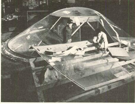
The oval shaped acrylic dome has an elliptical base with a 27-ft major axis and a 19-ft minor axis; height is 6 ft. It was formed from 10 side sections and one top section, bolted together on ½- by 1-in. plastic ribs
