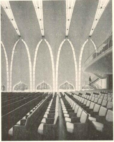
The skylights are equipped with interior amber glass bottom diffusers to reduce sun glare. The top exterior surfaces are glazed with opal glass. For nighttime lighting a combination system of dimmer-controlled incandescent and fluorescent lighting has been installed within the skylight construction between the inner and outer panes of glass. Lighting accents are provided by leaded glass panels in the end and side walls
