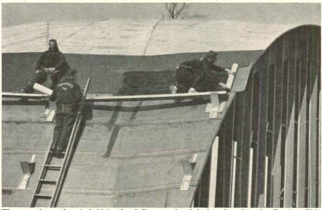
The one-ply roofing is laid in the full coat of polyisobutylene-based adhesive. Side laps of the roofing are 3 in. wide while end laps are 6 in. wide
