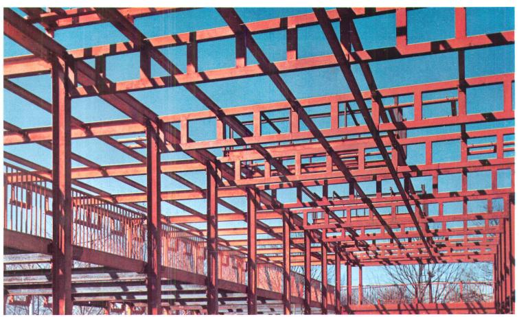
In Vierendeel trusses used to support roof, monorails, and mechanical equipment, hollow structural sections provide clean architectural appearance. Structurally economical for medium spans. Ductwork and piping can be routed through truss panels. Used at Guggenheim Laboratories, Princeton University to obtain maximum flexibility in meeting continually changing requirements of laboratory duct systems. Architect: Scrimenti, Swackhamer & Perantoni, Somerville, N.J.
