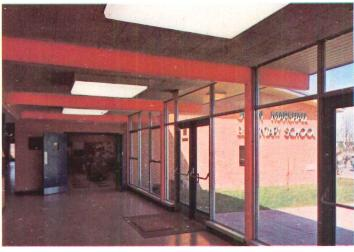
Beam and column assembly of hollow structural sections uses structural elements as window mullions. Beam is cantilevered to provide a sunshade and entrance cover. Architect: Scrimenti, Swackhamer & Perantoni, Somerville, N.J.
