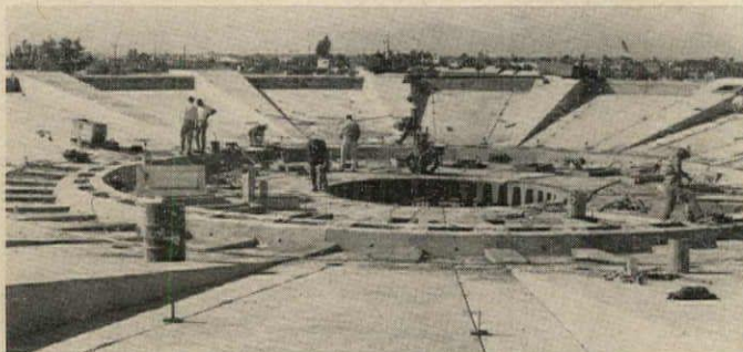
Above left: Close-up of tension ring shows both radial and longitudinal post-tensioning cables. Above right, top: High-hat double tee unit is ready to be hoisted in place; note post-tensioning cables at end and precast section of compression ring on the side. Above right: Shallower double tee being lifted to a position atop column arms
