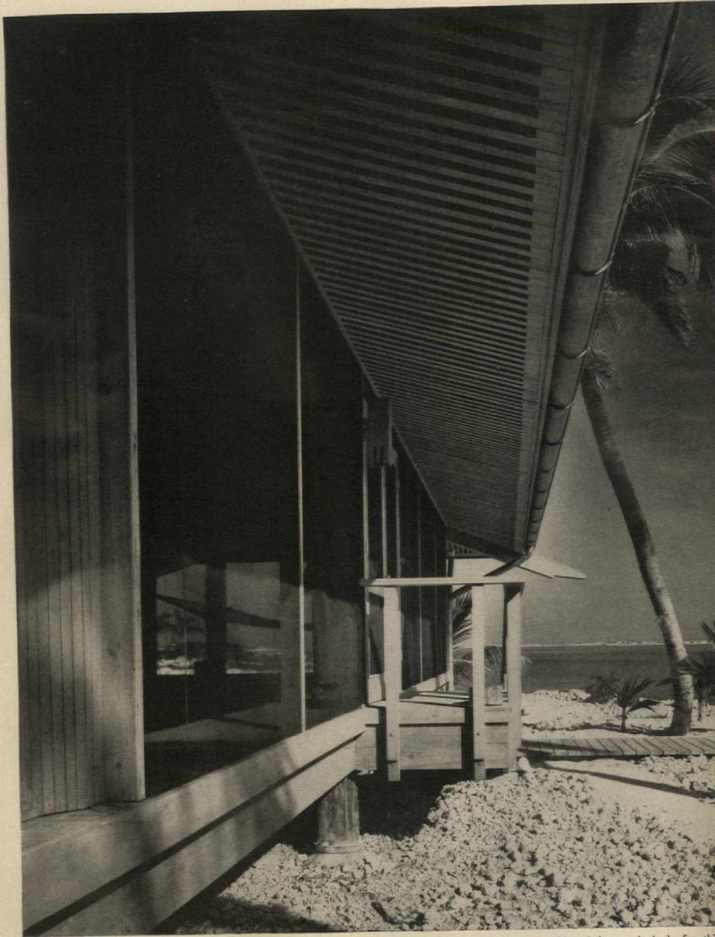
Graceful overhang provides shelter and shade for this Florida home. Pole construction withstands winds and water. Architect: Robert B. Browne, A.I.A., Miami, Fla.
