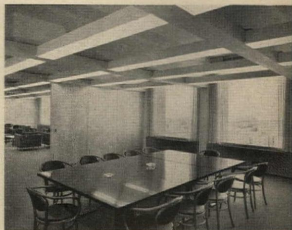
Above: A typical laboratory, corridor and seminar arrangement. Troffers alternate with beams for corridor lighting
