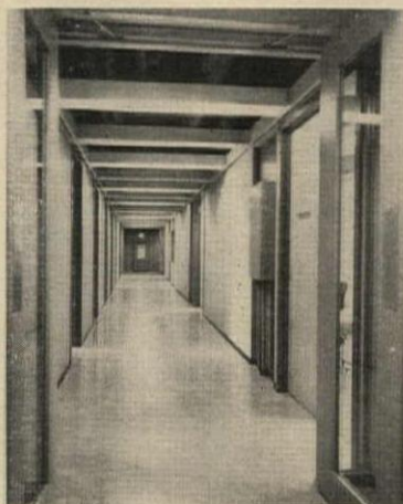
Above: A typical laboratory, corridor and seminar arrangement. Troffers alternate with beams for corridor lighting
