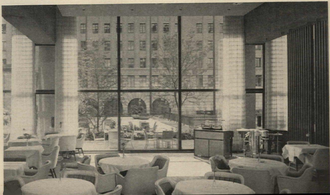
Restaurant at plaza level
