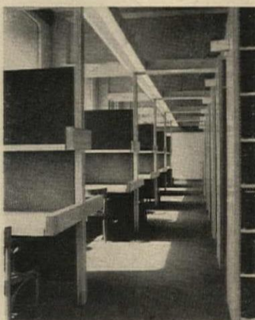
Above: The library, library carrels and auditorium. Adjustable acoustical reflecting panels occupy spaces between girders
