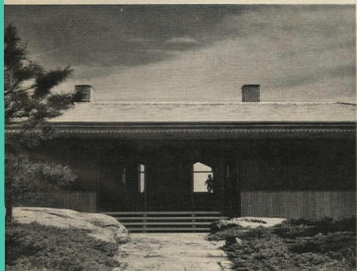
Landscaping of Residence in Greenwich, Connecticut Landscape Architect: Arthur Edwin Bye Jr. Architect: Ray Johnson
