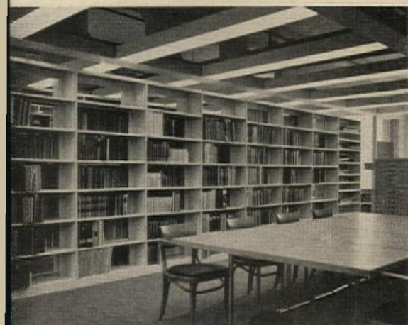
Above: The library, library carrels and auditorium. Adjustable acoustical reflecting panels occupy spaces between girders
