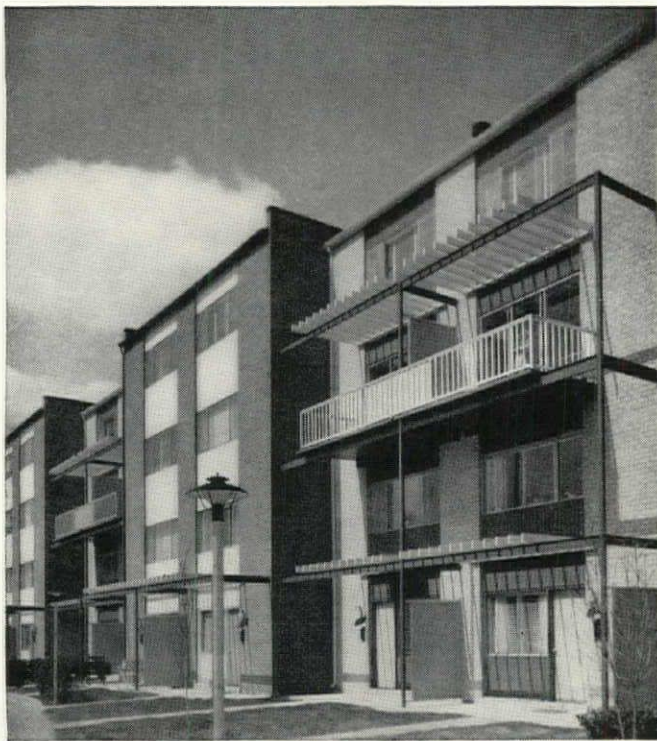
Fairview Associates' Town Houses, West Hyattsville, Md. Stearman & Kaplan, Bethesda, Md., Builders
