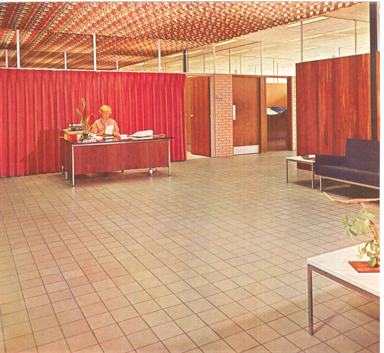
Robert E. Lamb, Inc., Valley Forge, Pa. Murray quarry floor is 6" x 6" x 1/2", Fawn Gray. Architect: Jules Gregory. Tile Contractor: Wissahickon Tile Company. Plate 510.
