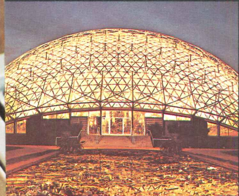
By lighting entirely from within, Westinghouse floodlighting is used in an artistically unusual way. Effect is heightened by revolving light shields of red, blue, yellow and white.
