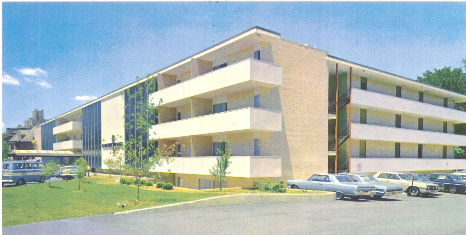
Parkway House Hotel, St. Louis, Mo. Architects: J. Richard Shelley, Robert P. Zamboni and Associates, Long Beach, Calif. Owned by: Rosenblum Construction Company, St. Louis, Mo.
