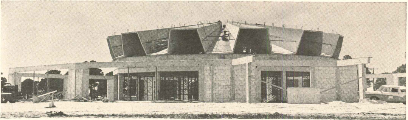
At St. Ambrose School and Provisional Roman Catholic Church, schoolrooms surround the religious area which is located under
