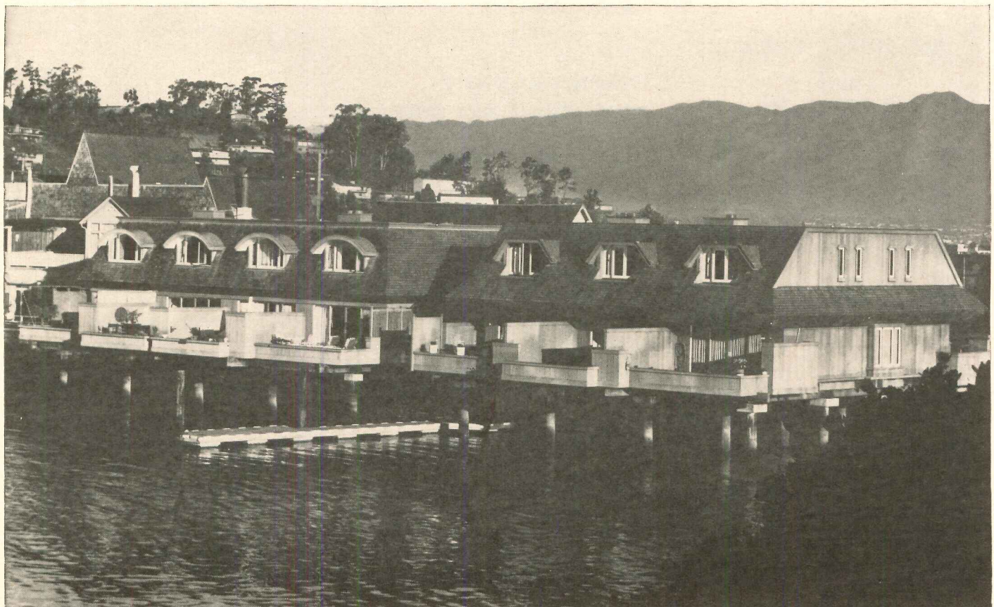
Wood, first wedded to water by early shipbuilders, goes modern with today's homebuilders. Pole construction of the Cove Apartments in Belvedere, California, withstands wind and weather. Owner: Belvedere Land Company. Architect: Charles Warren Callister,
