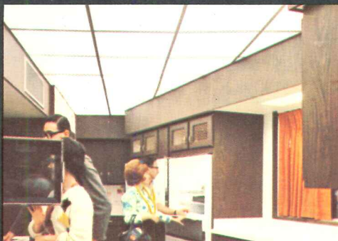
Luminous ceiling brightens kitchen. Westinghouse Stripliner luminaires are installed above plastic panels. Panels easily removed for simple lamp replacement and cleaning.
