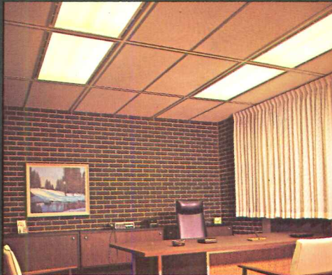
New Westinghouse Colamar Mark 50 controls air, acoustics and lighting in one space-saving ceiling system. Flexible to fill individual requirements and to give complete design freedom.
