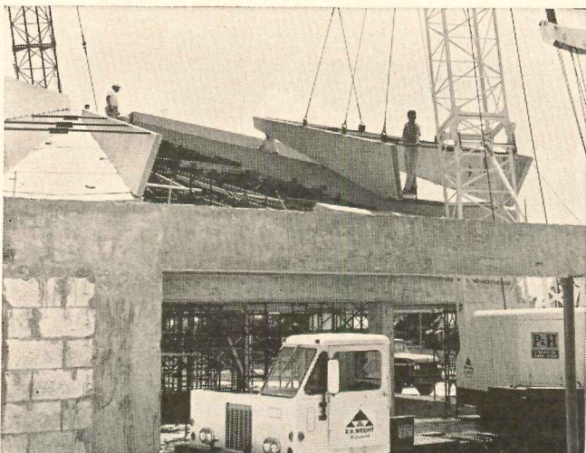
(LEFT PHOTO) Placing one of the 36' long precast concrete tapered folded plates. Only two days were required to place the 24 roof units. (RIGHT PHOTO) Deep folded plate design is
