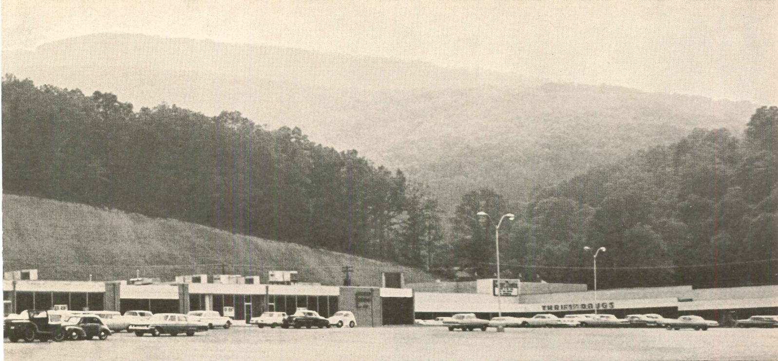
Searstown, Cumberland, Maryland. C. Yoder & Sons, Heating and Cooling Contractor.
