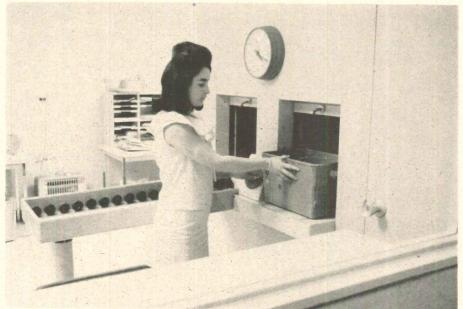
A service mail room on the 15th floor of the Penney building. Trays are dispatched on the right and delivered on the left; the floor selector is between the hatches.
