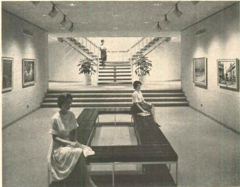
In addition to the studio areas on the platforms, the building provides a variety of galleries for display of painting and sculpture. Interior wall surfaces are painted concrete or block, or plastic covered gypsum board. Floors are covered with carpet or composition.
