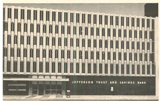
A light stainless steel clad facing grid supports a decorative pattern of stainless steel panels on this remodeled bank. A background screen of black porcelainized expanded metal hides the old surface and adds deep dimension.
