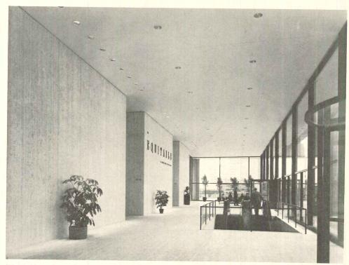
The lobby, above, has walls and floor of travertine marble; is enclosed by large sheets of clear ½-inch plate glass set in frames of aluminum with a hard anodic black coating. The conference room pictured below is part of the Equitable executive complex
