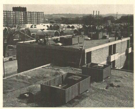
Sale town houses each have their own roof-mounted condensing units. Below left, A 750-ton hermetic centrifugal unit in the basement of one of the high-rise buildings provides chilled water for air conditioning the rental units. Below right, Gas fired furnaces in the basements of the sale town houses are equipped with cooling coils which are connected to the roof-top condensing units.
