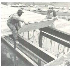
Handling of the DUAL TEE System takes a minimum of time and effort. The relatively light-weight INSULROCK tiles go down fast in the hands of experienced, franchised applicators.
