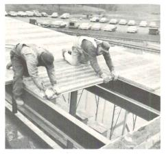
Fitting one tile snug up to adjoining tiles is a snap with the new DUAL TEE System. And the roof deck is one flat, smooth surface, eliminating any need for grouting.
