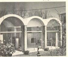
1964: I. M. Pei creates arches of bearing brick and poured concrete.
