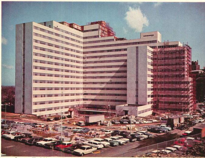
Over one million bricks were replaced by Plasteel aluminum panels while the hospital continued its day-to-day operation.
