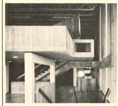
A concrete skeleton system was used in the lower level with exposed steel pan floor and roof construction. Contained in this section are spectator seating, locker rooms, offices, classrooms, custodial areas, and swimming pools.
