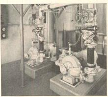
Typical installation photo of a Uni-Pressure System illustrates the compactness of a type II System. This equipment is designed to provide a maximum of 150 GPM and a system pressure of 83 psi.
