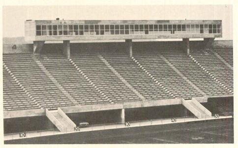
Modified Lin T's spanning 50 ft are arranged in an arc to improve sight lines. They are notched in the center to allow for steps, and have diaphragms at the ends to prevent tipping. The diaphragm is shown in section A-A, notching of the T in section B-B. The diaphragm and web of the T are supported on poured-in-place walls as shown in the drawings at bottom of the page. Photo was taken before wood seats were installed.
