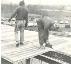
Spot weld the support member to the subpurlin and the DUAL TEE unit is secure - a virtually solid system of interlocked supports and tiles.
