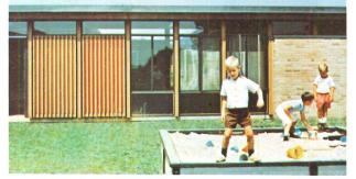
Glasweld's remarkable freedom from maintenance makes it practical for you to use color freely in out-of-reach places such as these orange and yellow panels mounted behind pressure-treated 2 x 3's. A simple hosing down is the only maintenance these and the adjoining black Glasweld sandwich panels will ever need.
