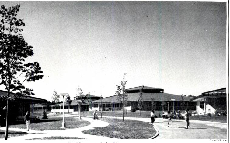
All buildings-except the hospital which is reinforced concrete—are steel frame with brick cavity walls and poured concrete floor slabs.
