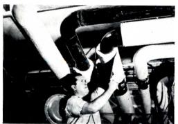
reduced by age, moisture or humidity, as can happen with chemically treated barriers. 2. Pyro-Kure meets the standards for non-combustibility of the National Building Code and has been approved by the Board of Standards and Appeals of New York City. 3. Pyro-Kure has a minimum MVT rate for maximum protection against condensation damage to insulation.
